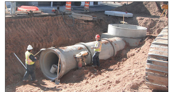
Storm Sewer Installation
