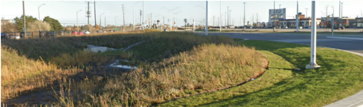
Bioretention area that provides additional water quality treatment
