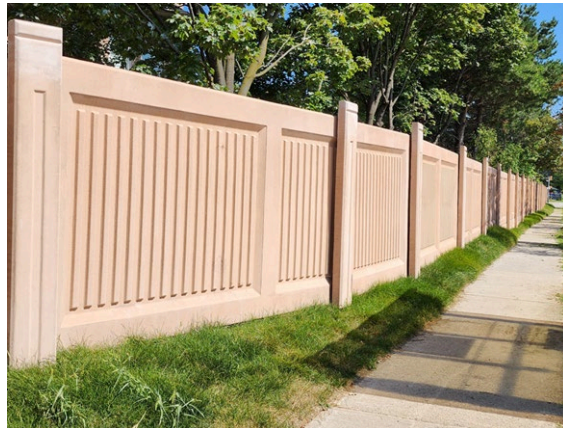
Mississauga Standard Concrete Noise Wall
