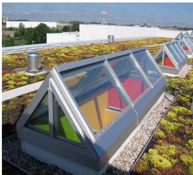
Figure 9-38: Green roofs are an effective stormwater best management practice and contribute to the reduction of the urban heat island effect.
