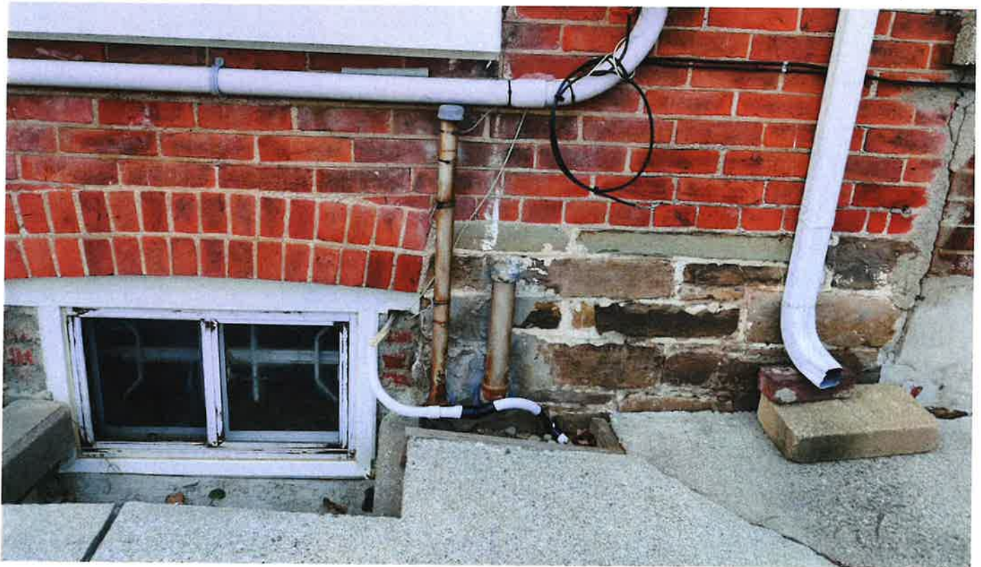
General view of the filler for the AST in the basement (looking South)
