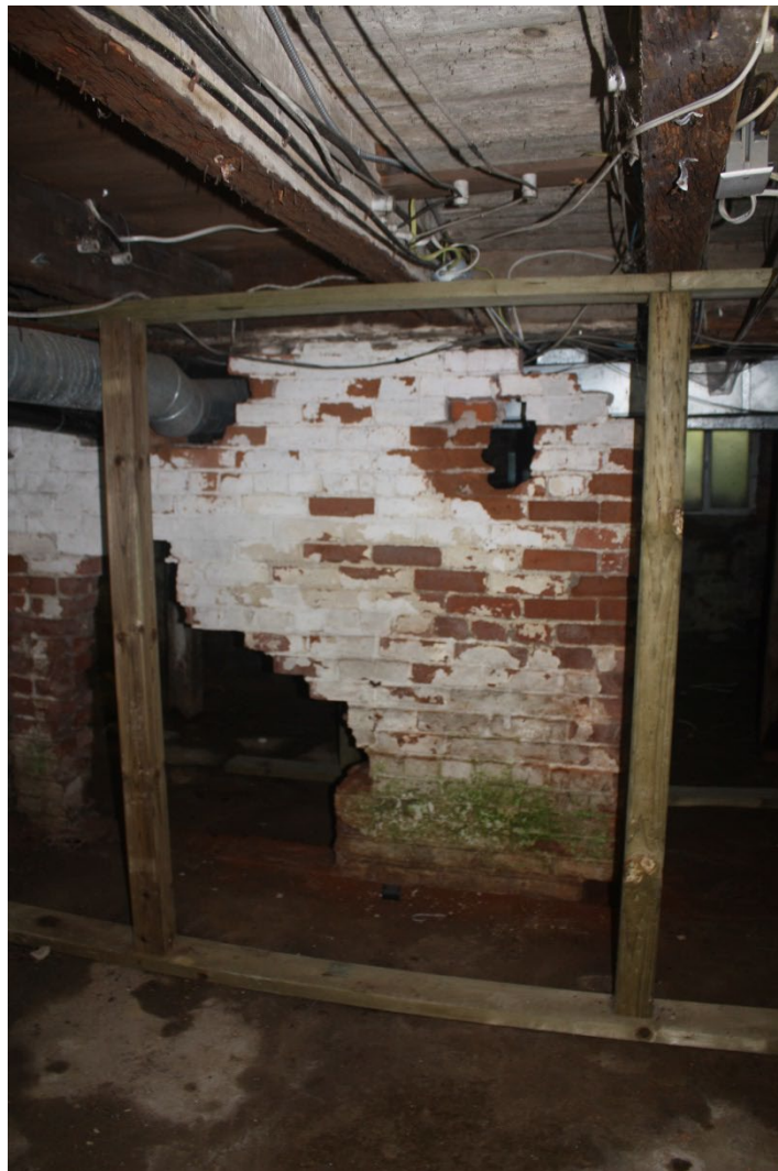
Figure 75 A gap in the interior basement wall of the original farmhouse and supporting timbers, 2013 (Photo by author.)
