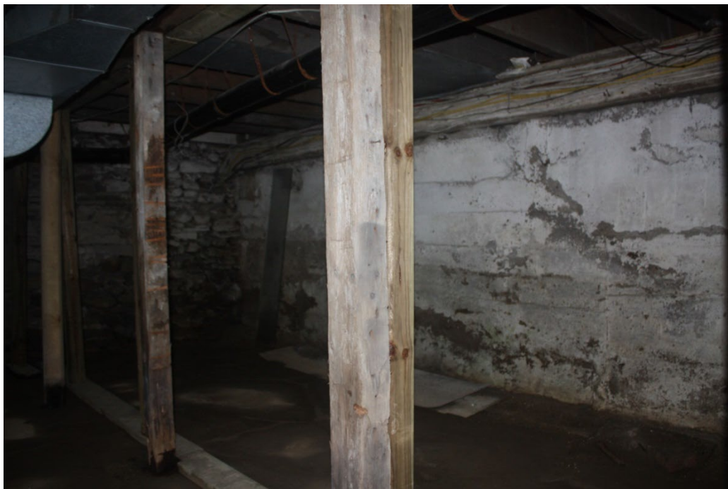
Figure 73 The basement of the addition, 2013. Timber had been inserted to support the structure (Photo by author.)
