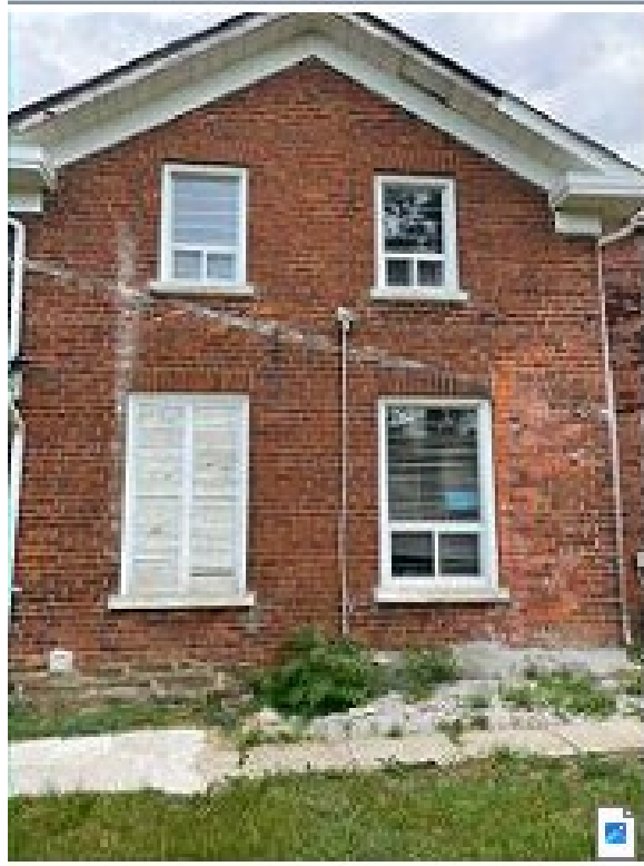
Figure 33 Detail of the west façade, 3650 Eglinton Avenue West, showing the returned eaves and window treatment, 2023 (Photo by owner.)
