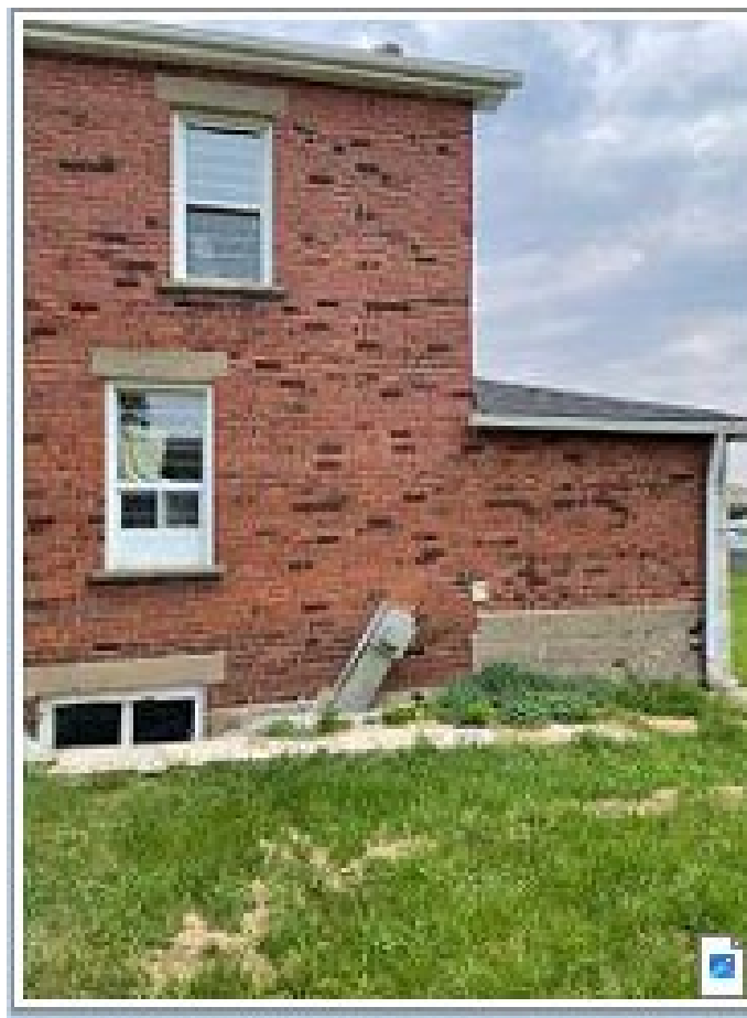
Figure 39 Continuity of brickwork on the west façade of the addition, 2023 (Photo by owner.)
