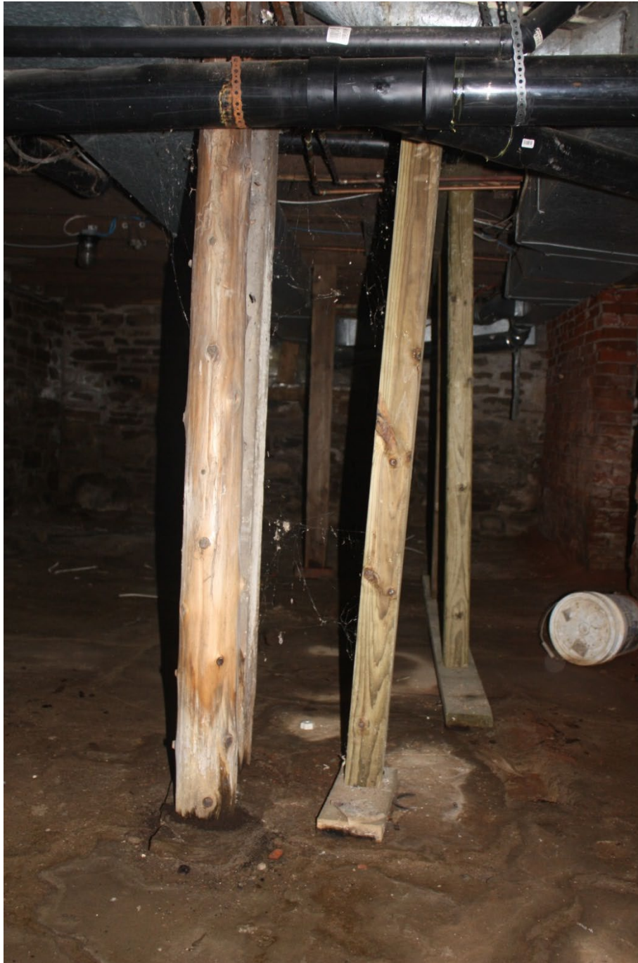
Figure 74 timber supports in the basement of the original farmhouse, 2013 (Photo by author.)
