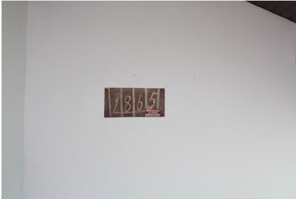
Figure 10 The interior north wall of the one storey addition, 2013. The wall board has been cut away to display a portion of the south exterior wall of the original dwelling. The vertical fan shape of the bricks here suggests that the date was placed on a window arch now hidden by the modern addition (Photo by author.)
