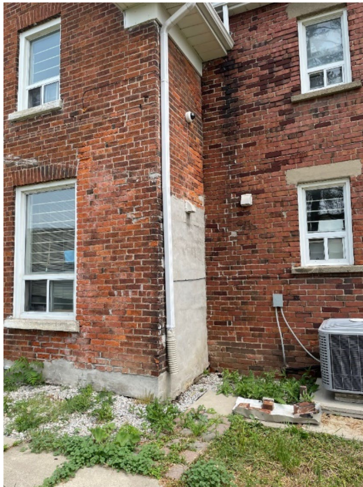
Figure 37 Deteriorating brickwork at the southwest corner of the original farmhouse, 2023 (Photo by owner.)
