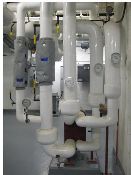
Figure 4: Typical ETS Installation
