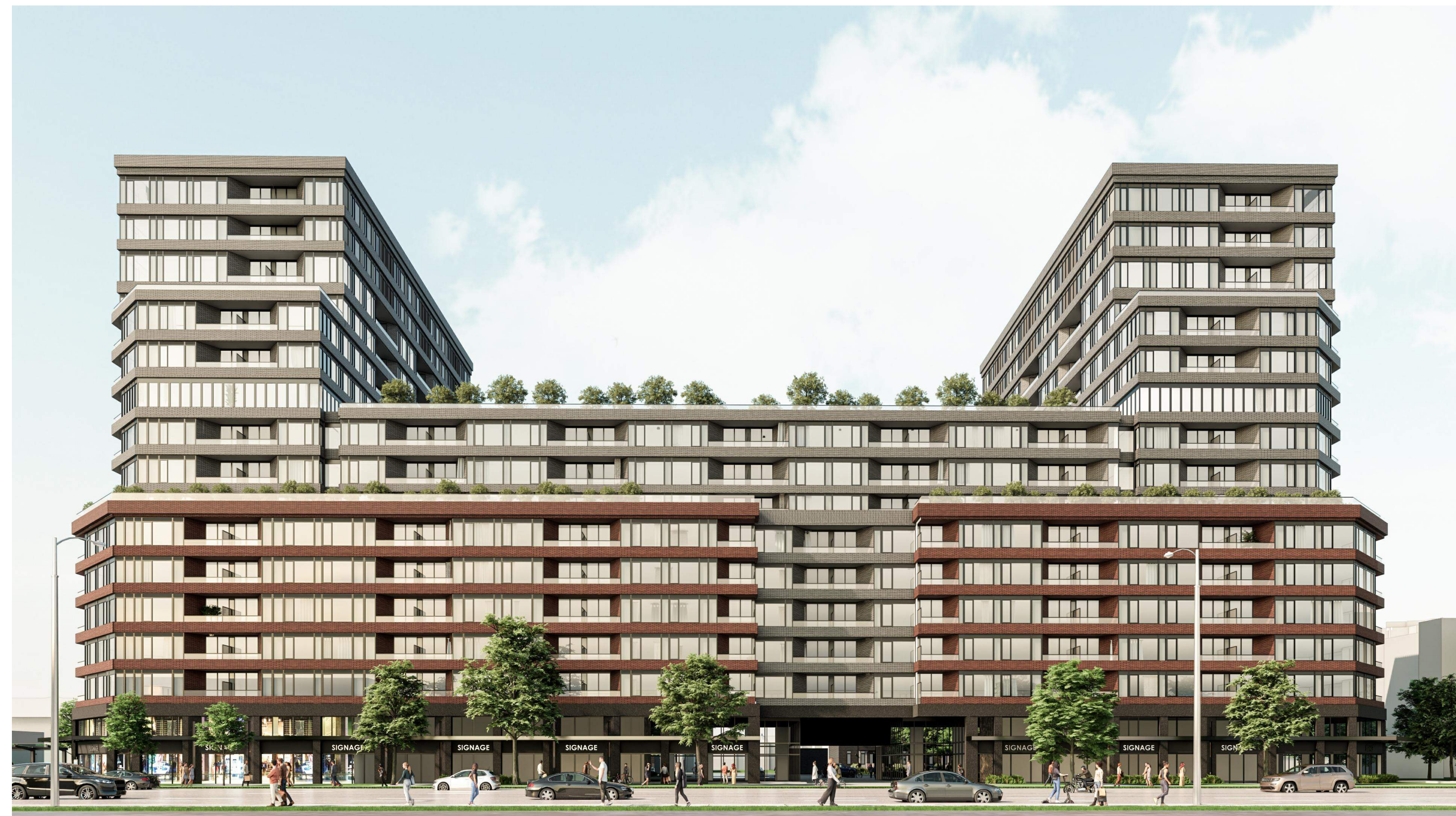
2. PEDESTRIAN VIEW LOOKING NORTH
