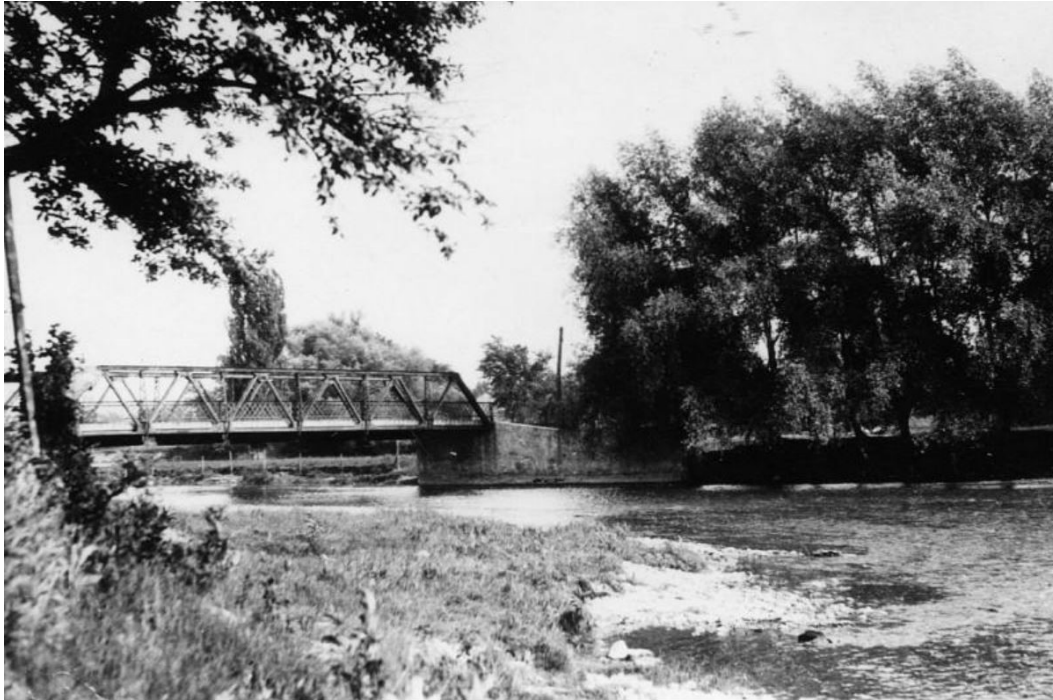
Figure 3-8: Derry Road Bridge over the Credit River, Meadowvale, photo is labelled c1920 however the photo likely postdates 1930 as this is the date of construction of the bridge (Heritage Mississauga)
