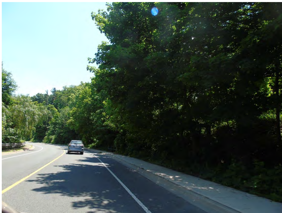
Figure 11-18: Mississauga Road, south of Dundas Street (A.S.I. 2018)
