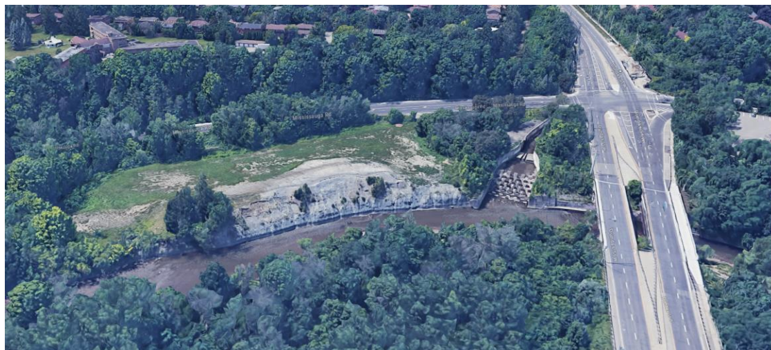
Figure 3: The bank of the Credit River at the subject property with the Sawmill Creek flume channel immediately to the right, followed by the Dundas Street bridge over the Credit River (Google Maps, 2026)
