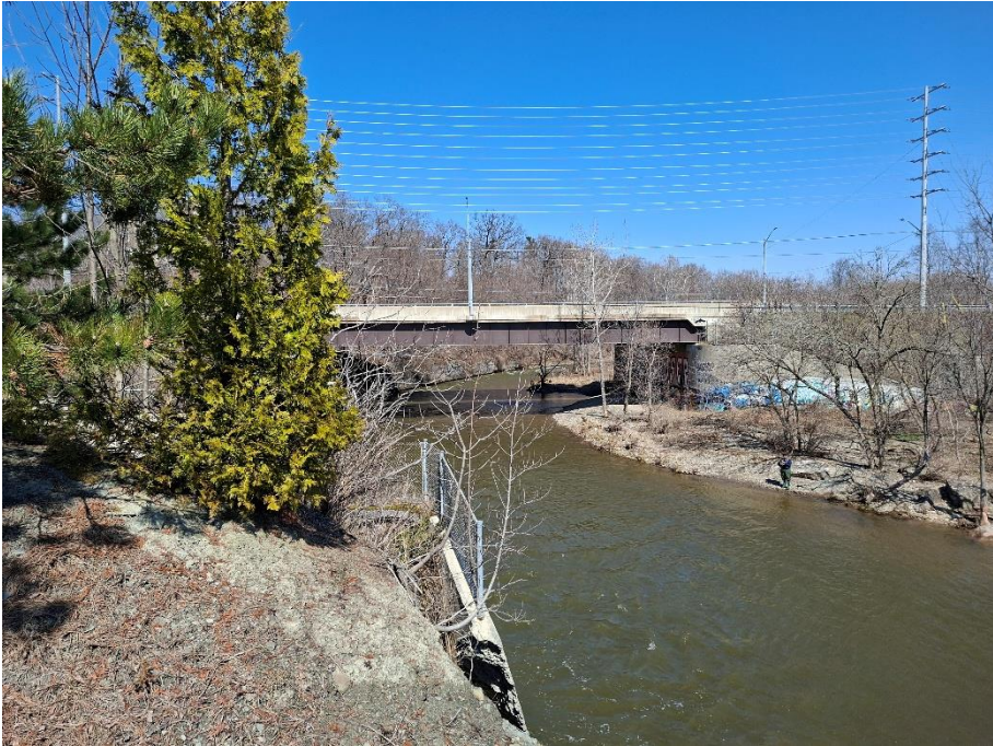
Plate 36: The Dundas Street West Bridge, view from the subject property (A.S.I., 2026)
