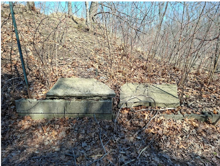
Plate 24: Concrete previously part of a garage at the subject property (A.S.I., 2026)
