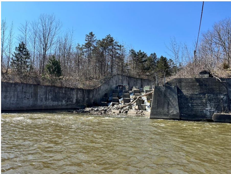
Plate 5: Sawmill Creek flume channel viewed from across the Credit River (A.S.I., 2026)
