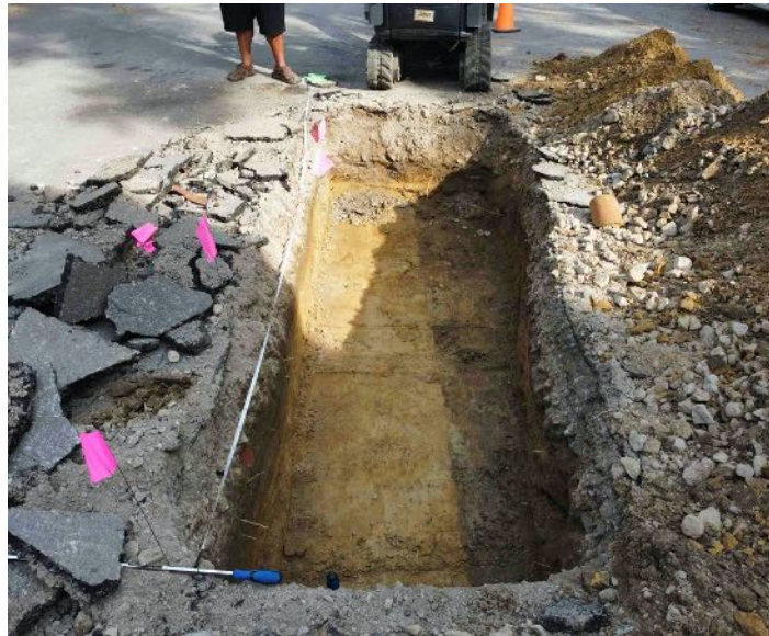
Plate 5 Shows Stage 3 trench excavation - main drain.
