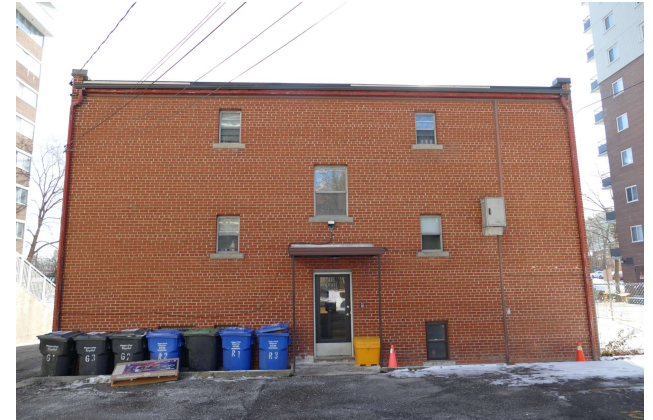
P3 - North Elevation of the Subject Building
