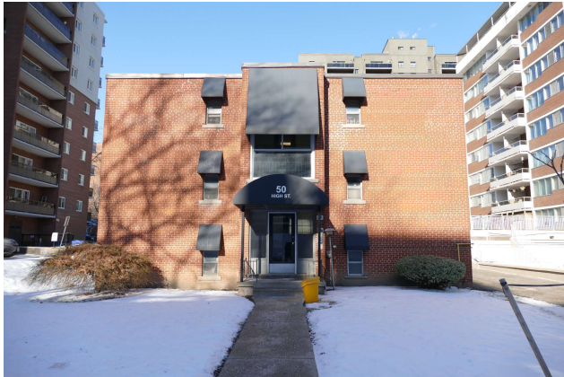
P1 - South Elevation of the Subject Building
