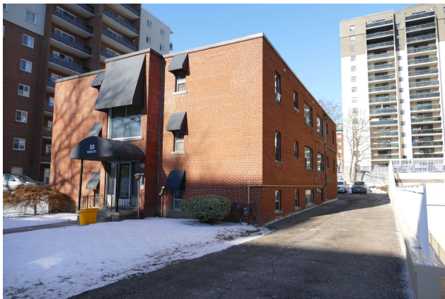
P4 - East Elevation of the Subject Building
