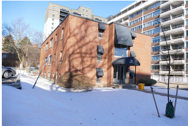
P2 - West Elevation of the Subject Building
