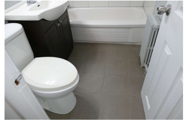
P9 - Typical Bathroom Within the Apartment Units
