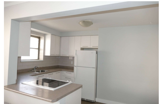
P6 - Typical Kitchen Area Within the Apartment Units
