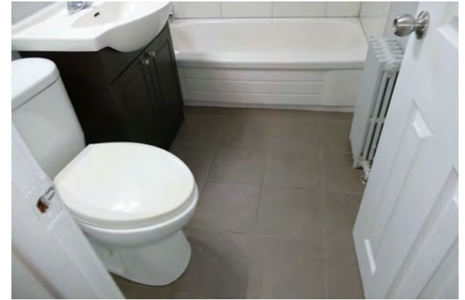
P9 - Typical Bathroom Within the Apartment Units
