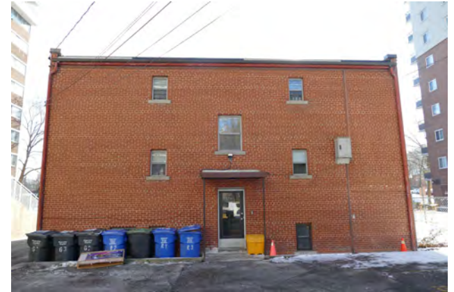
P3 - North Elevation of the Subject Building
