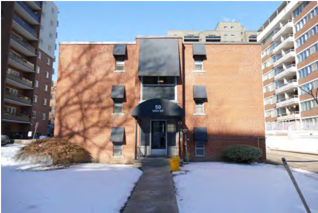
P1 - South Elevation of the Subject Building
