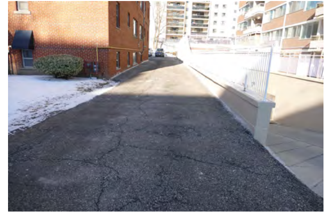
P15 - Asphalt Paved Driveway on the East Portion of the Site
