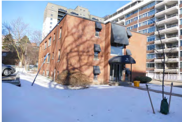
P2 - West Elevation of the Subject Building
