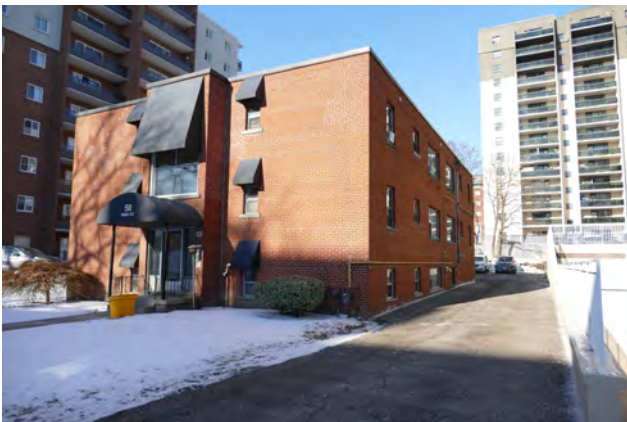
P4 - East Elevation of the Subject Building
