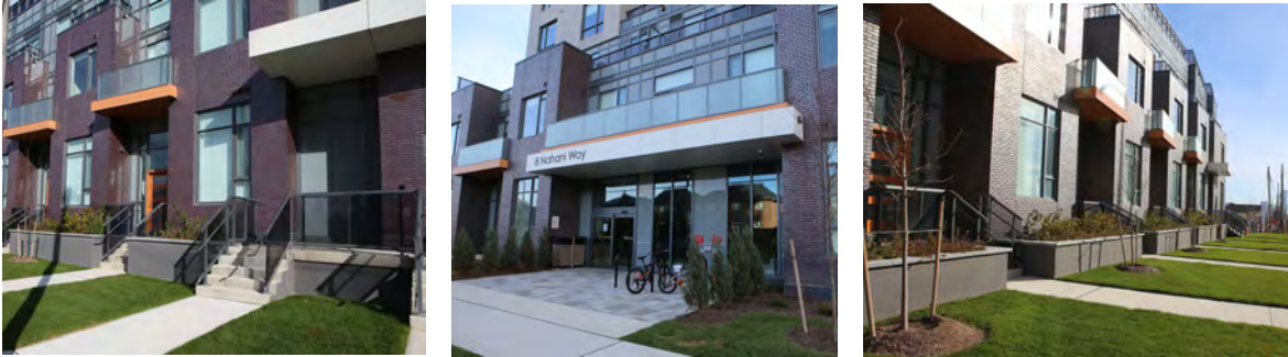
Examples of Wind Mitigative Measures at Entrances (recessed entrances, railings, canopies, raised planters, coniferous trees).
