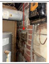
**Photo #6:** Chimney cleanout located behind the present day forced air furnace and hot water heater in 66 Agnes Street (indicated by red arrow).
