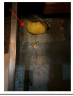
**Photo #4:** Foam-filled historic location of vent and fill pipes within the present-day furnace room of 60 Agnes Street (indicated by red arrow).
