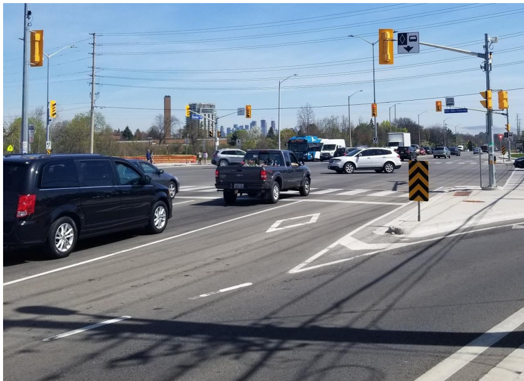
Figure 3-3. Example of Intersection Improvements (Queue Jump Lane)
