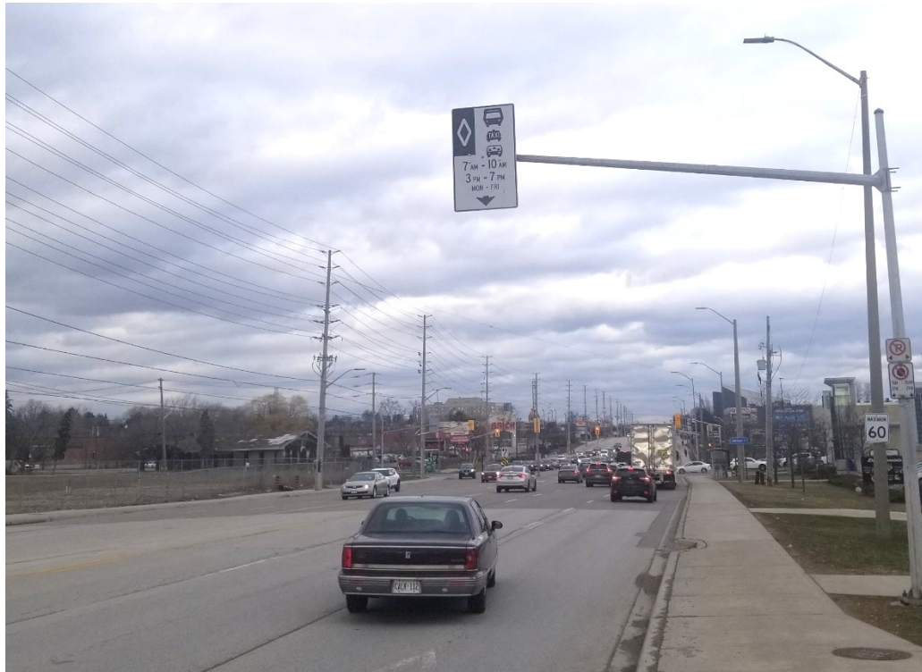
Figure 3-3. Example of Intersection Improvements (Queue Jump Lane)
