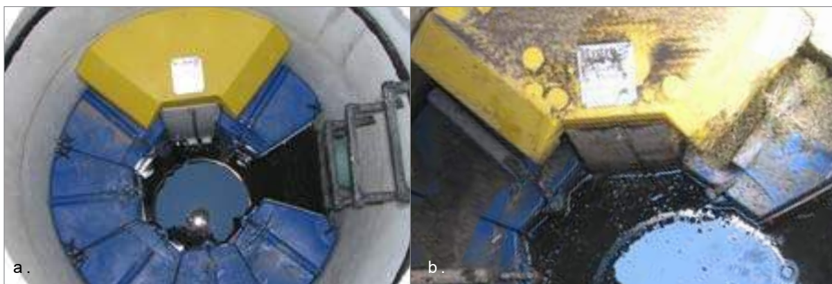
Fig.3 a) The water level in a properly functioning Up-Flo® Filter will drain down to the base of the Filter Modules. b) When the Drain Down Filter becomes clogged, the base of the Filter Modules will be submerged in standing water. Note, above right, that the Drain Down Filter is submerged in standing water.
