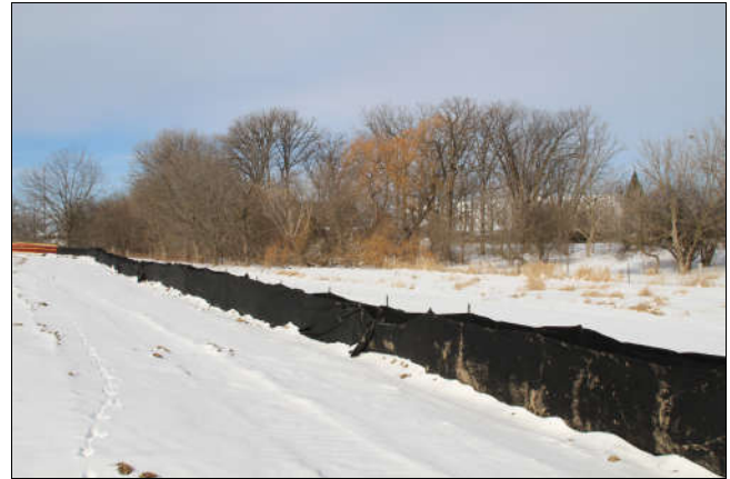
Figure 6 at property line at rear of proposed Data Centre
