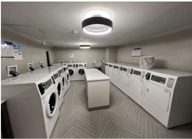
Photo 21: View of the laundry room in basement of Building B (1980 Fowler Drive), facing west.
