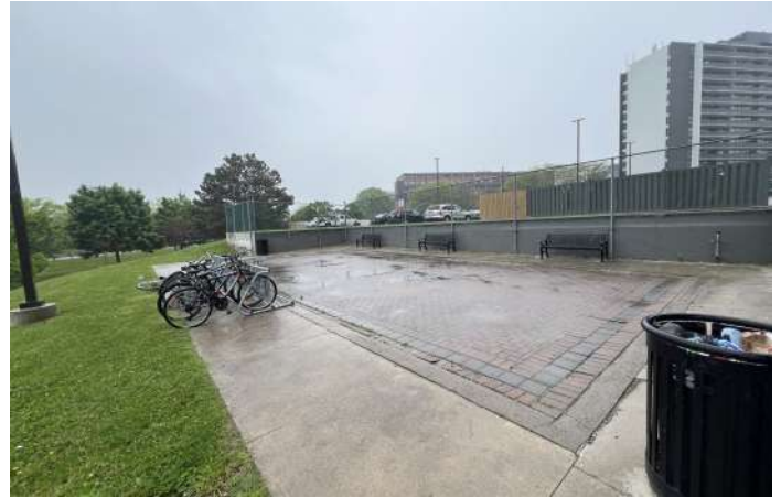
Photo 32: View of a former swimming pool east of Building B (1980 Fowler Drive), facing east.
