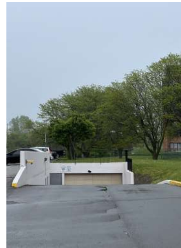
Photo 34: View of the underground parking ramp of Building B (1980 Fowler Drive), facing south.
