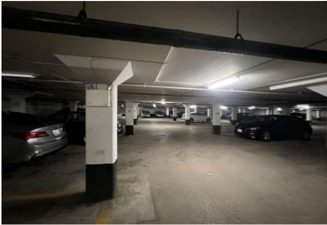
Photo 7: View of the underground parking garage in Building A (1970 Fowler Drive), facing northeast.
