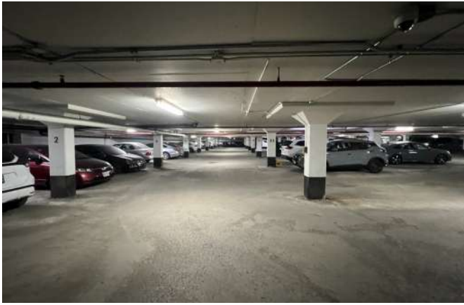
Photo 25: View of the underground parking of Building B (1980 Fowler Drive), facing northwest.
