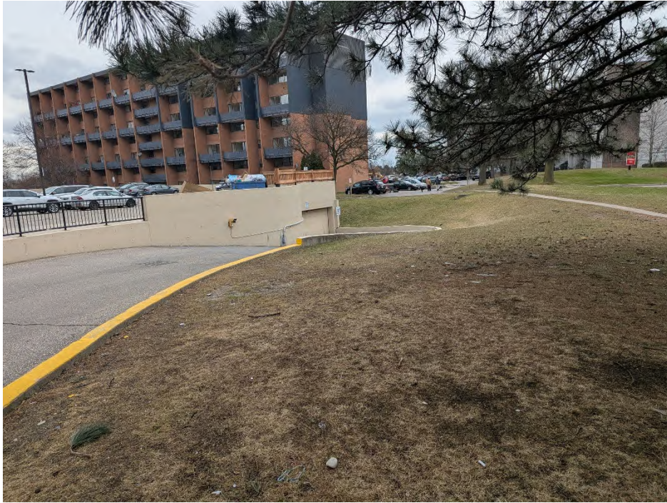
Image 7: View east to the ramp to the 1970 Fowler underground parking garage.
