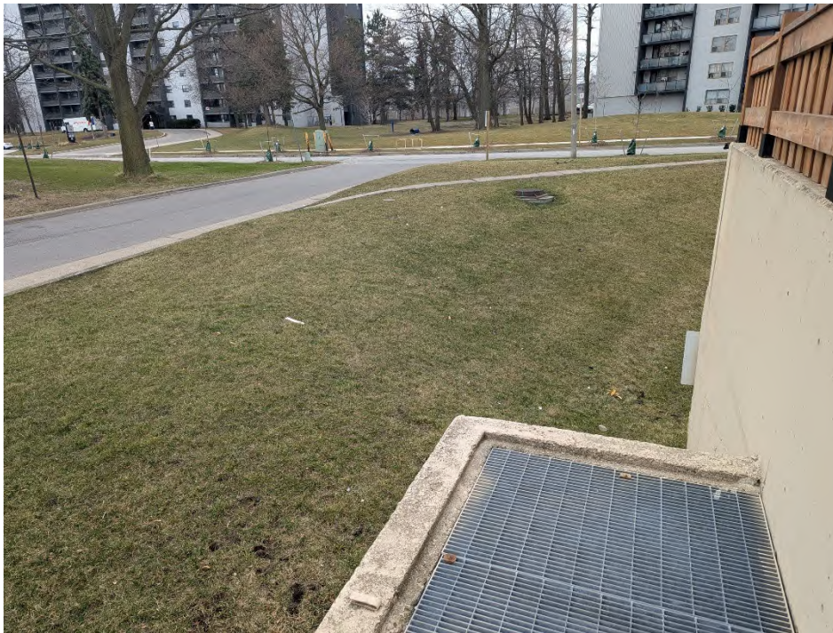
Image 6: View southeast near the entrance to the 1970 Fowler underground parking garage.
