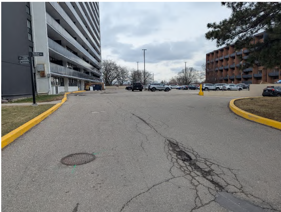
Image 8: View northeast along east side of the 1970 Fowler tower.
