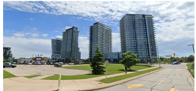
Image 3: View looking east at Subject Lands
