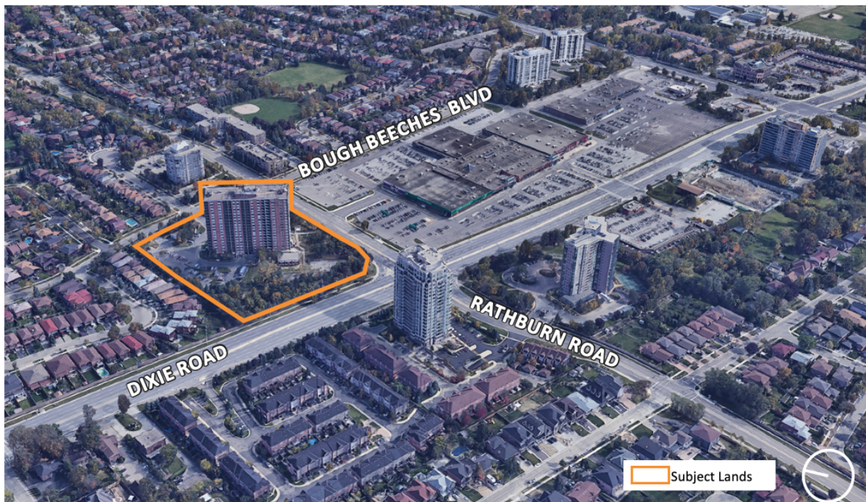
Figure 3: Oblique aerial view facing southeast
