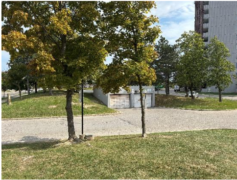
Image 3: Subject property, from northern corner, facing south.
