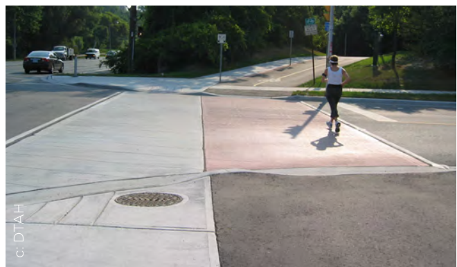
Figure 4.72. Crossroad markings and signs.
