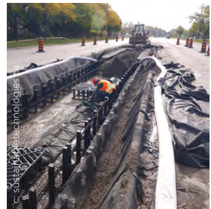
Figure 4.15. Soil cells (Central Parkway, Mississauga).
