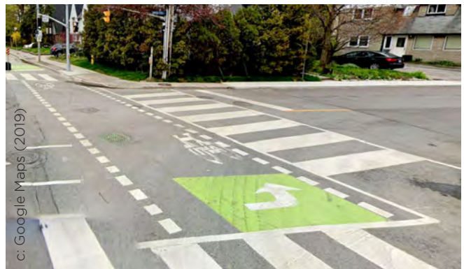
Figure 4.68. Signalized intersection with separated cycling facilities and bicycle two-stage left.
