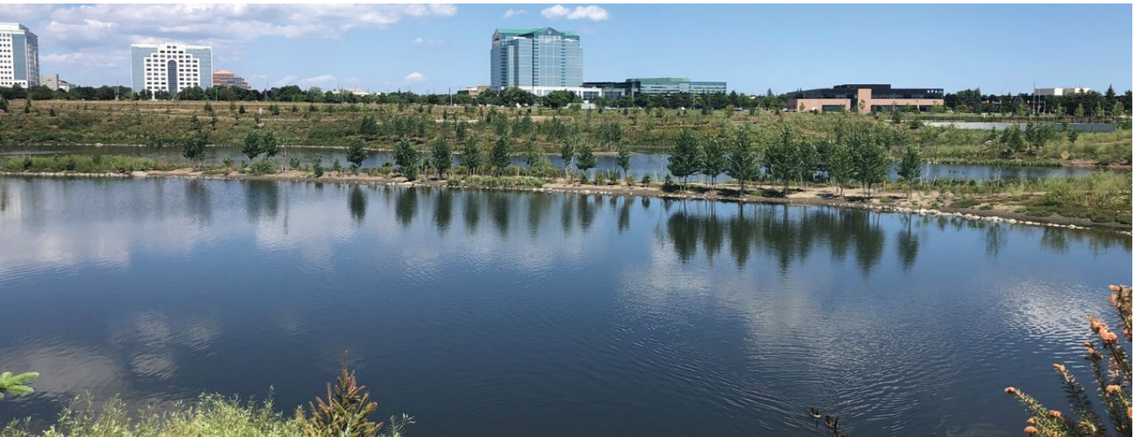
Figure 4.13. The Saigon Park stormwater management pond helps reduce the risk of flooding in the area and protects the water quality. (c. City of Mississauga )
