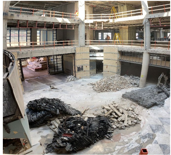
Figure 4.16. Construction waste diversion project for Hazel McCallion Central Library Renovation, where waste has been sorted in preparation for diversion. (c. City of Mississauga Staff)
