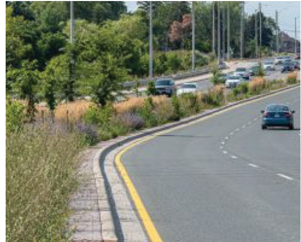
Figure 4.14. The bioswales along Mississauga Road represent the ongoing green infrastructure initiatives within the City. (c. City of Mississauga )
