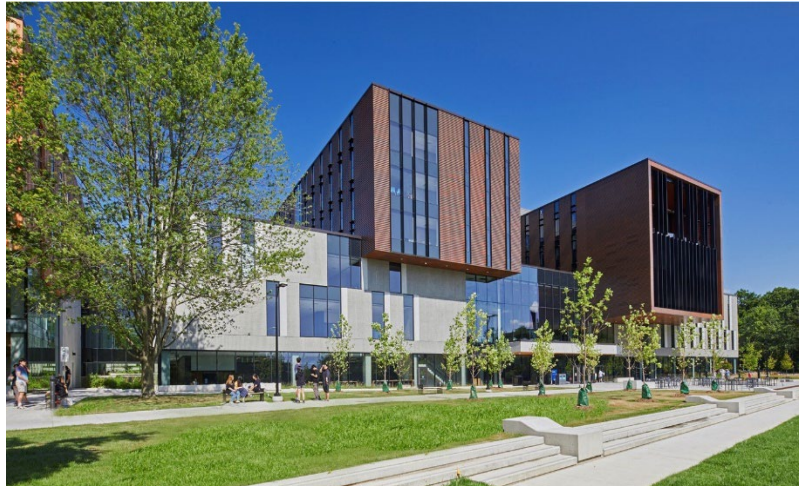
Figure 4.2. The Maanjiwe nendamowinan (2018) at the University of Toronto Mississauga, has an Anishinaabemowin name meaning “a gathering of minds”. This certified LEED Silver building features elements such as energy-efficient mechanical systems, a green roof space, and rainwater cycling. (c. City of Mississauga )
