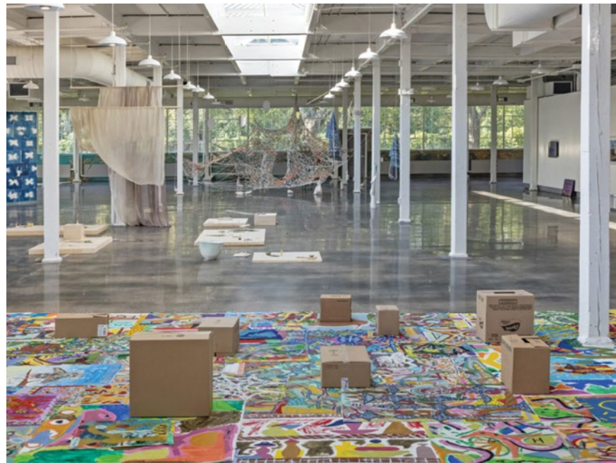
Figure 8.11. The Small Arms Inspection building, designated under the Ontario Heritage Act , has been renovated and transformed into a multi-purpose creative hub for the community. (c. City of Mississauga )
