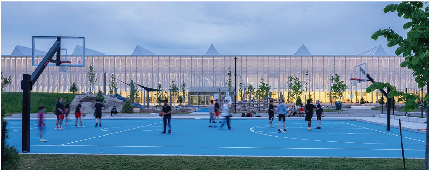
Figure 18.4. Churchill Meadows Community Centre and Mattamy Sports Park is a recreational facility equipped with a variety of amenities and programs. (c. MJMA Architecture & Design)
