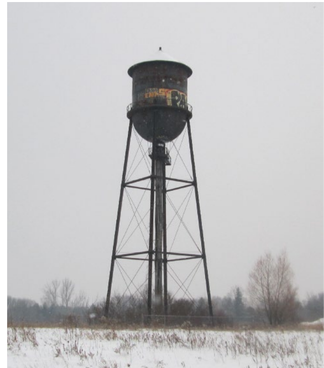
Figure 4. The Water Tower on the Canadian Arsenal Lands is one of the last remaining elements on these lands, dating back to 1910 (c. Hikina the GTA ).
