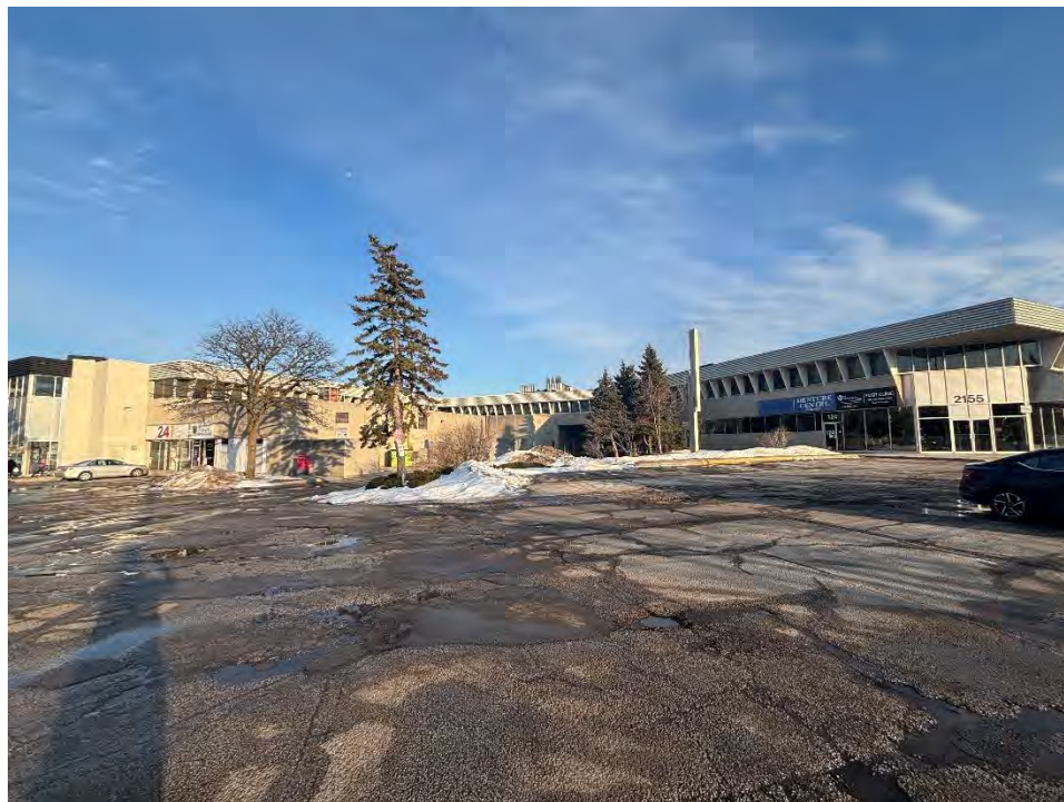
Photograph 2: View of a portion of the north elevations of Buildings A and B at the Property, looking southeast.
