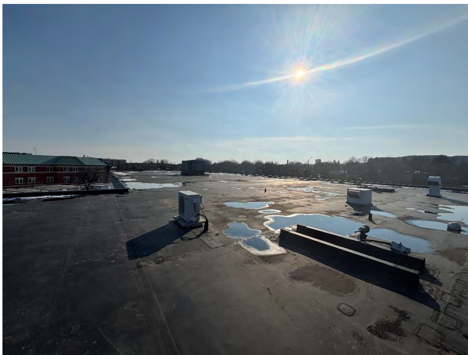
Photograph 22: View of the roof of Building B at the Property.
