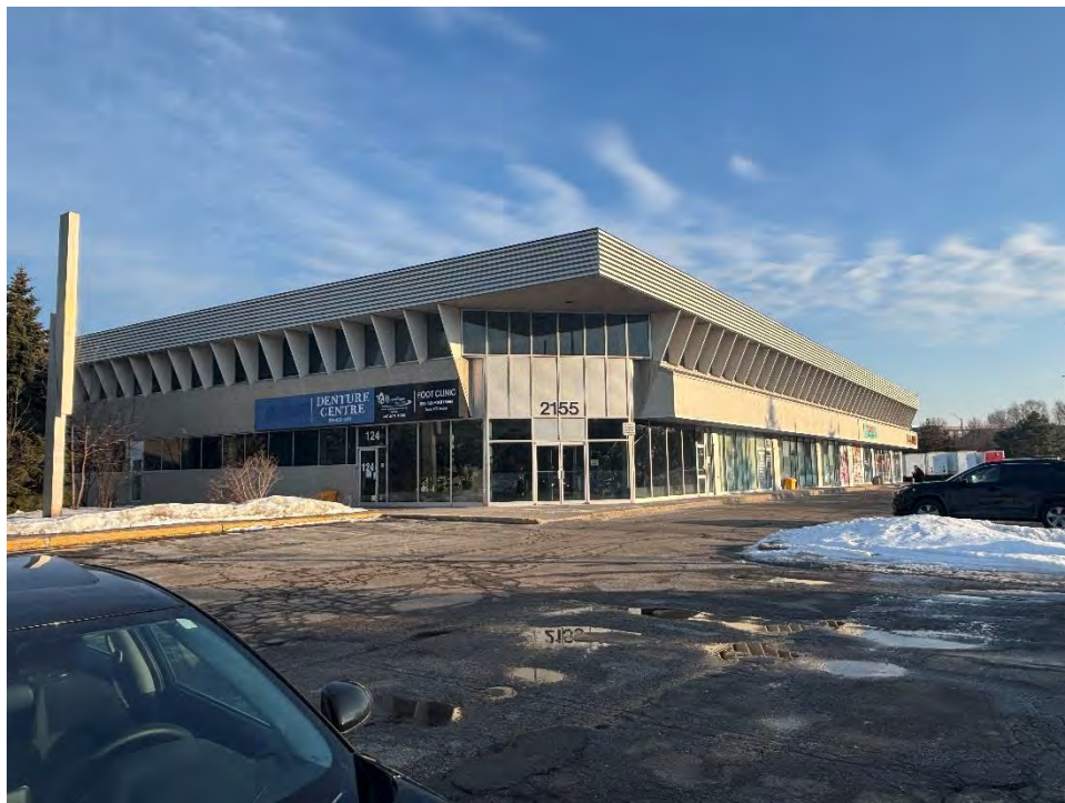
Photograph 1: View of a portion of the north elevation of Building B at the Property, looking south.
