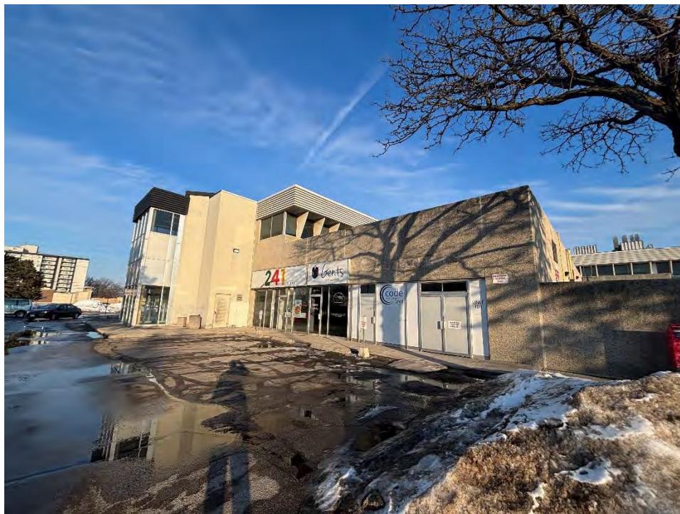
Photograph 3: View of a portion of the north elevation of Building A at the Property, looking south.
