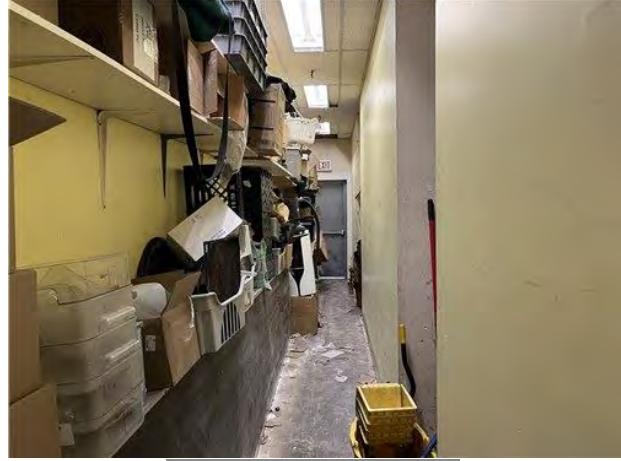
Rear Fire Exit Corridor
