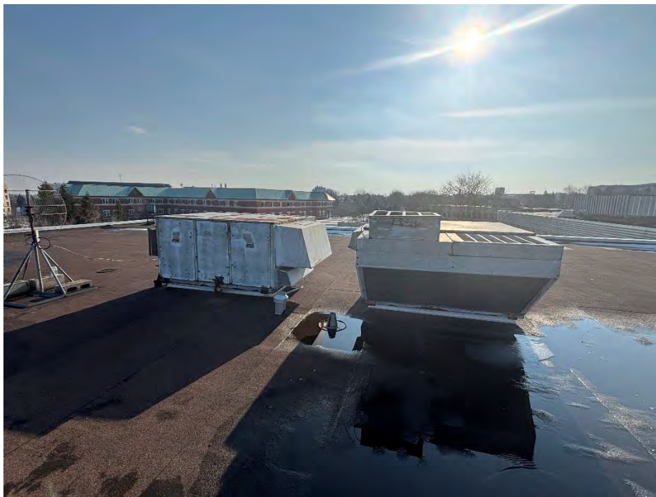
Photograph 23: View of the upper roof of Building A at the Property.
