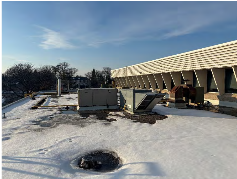
Photograph 21: View of the lower roof of Building A at the Property.
