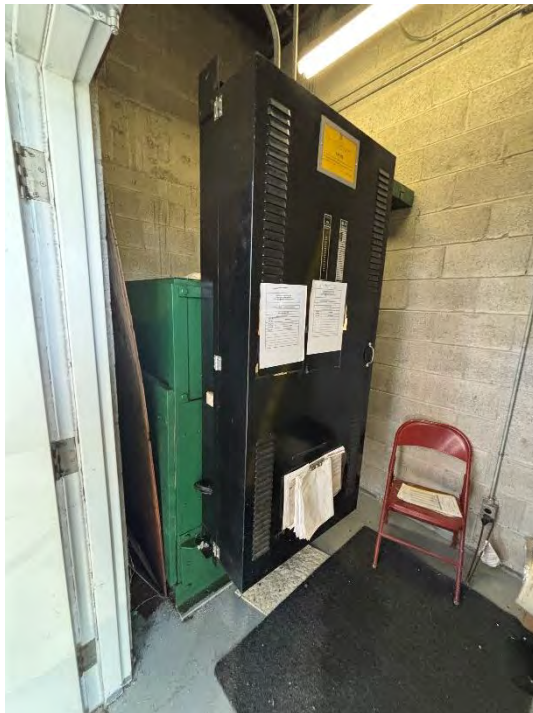
Photograph 25: View of the elevator room on the ground floor of Building B at the Property.
