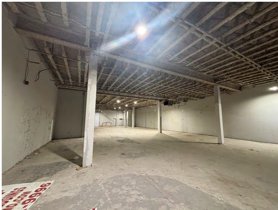
Photograph 17: View of Unit 107 (vacant) located on the ground floor of Building A at the Property.
