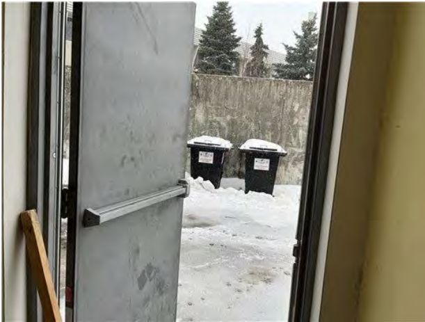
Rear Fire Exit Door
