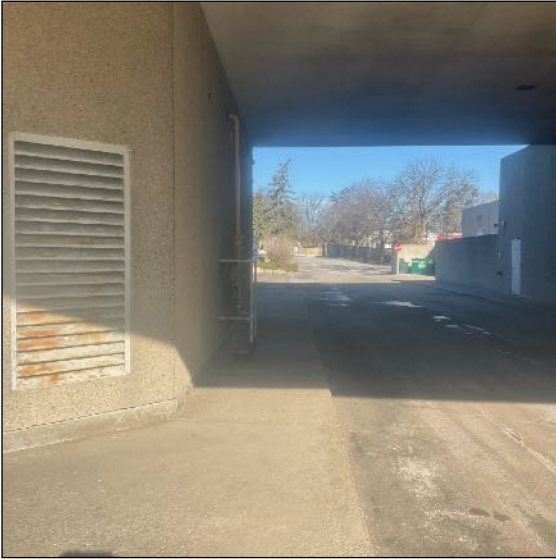
Image 5: Gas utility within Study Area.
