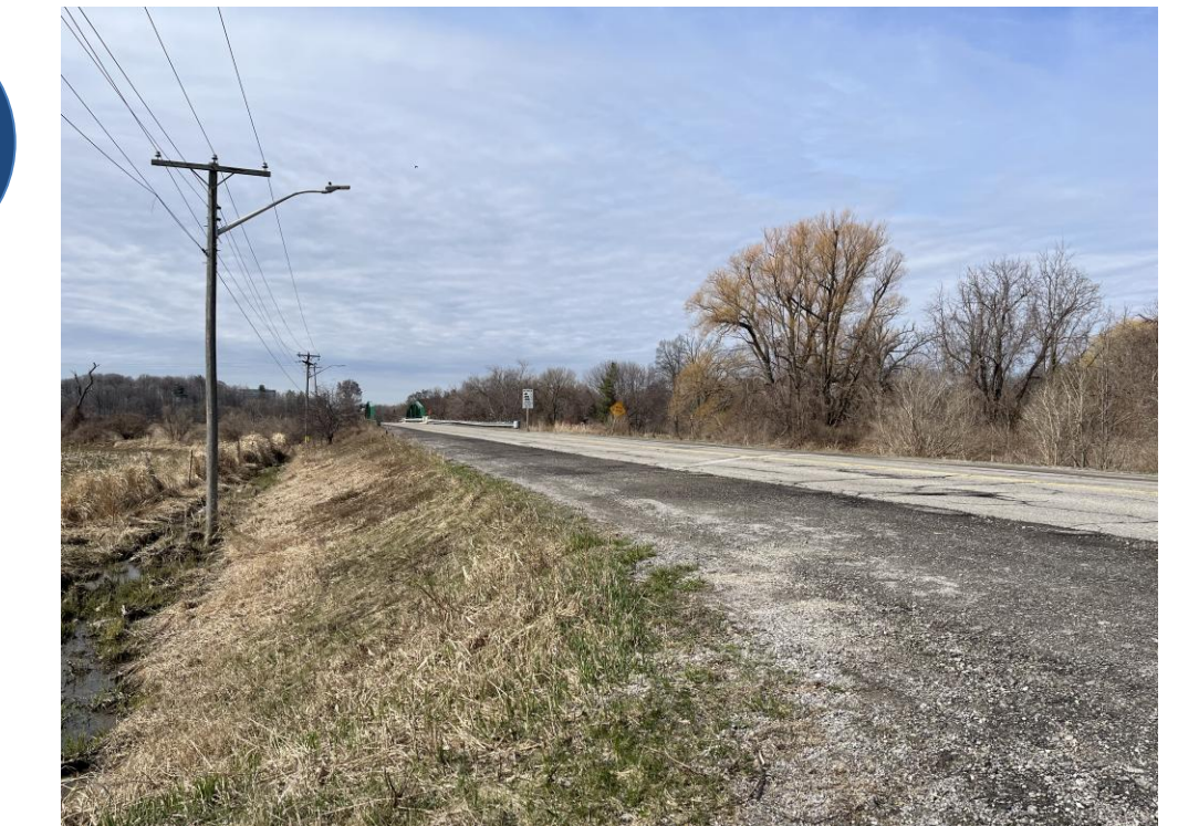
Sanitary trunk sewer installation on Old Derry Rd & Old Creditview Rd (Region of Peel)
