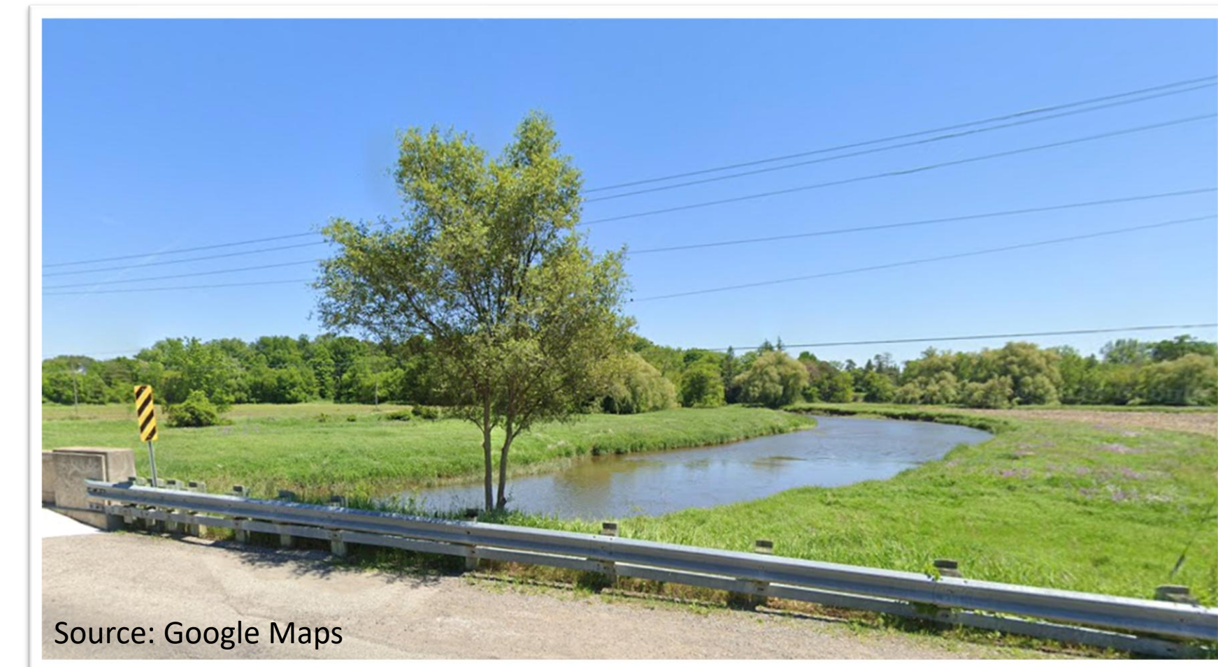
Credit River Watercourse Crossing
