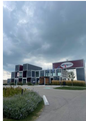
Picture 10: View of Mattamy's sales centre at the north adjacent property, facing north
