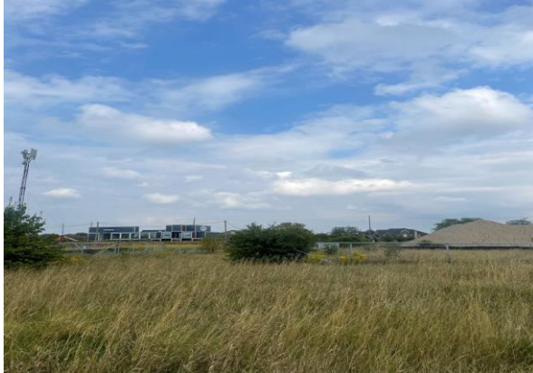
Picture 7: View of southern portion of the Site, and grading work at the south adjacent property, facing south.
