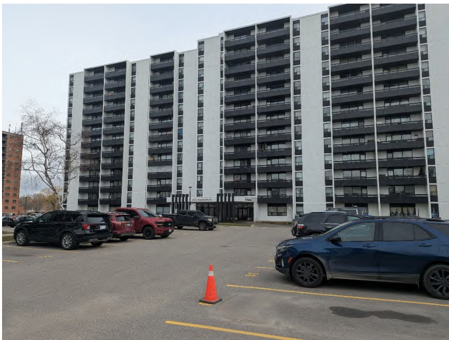
Image 2: View northeast across surface parking to the 2233 Hurontario building.
