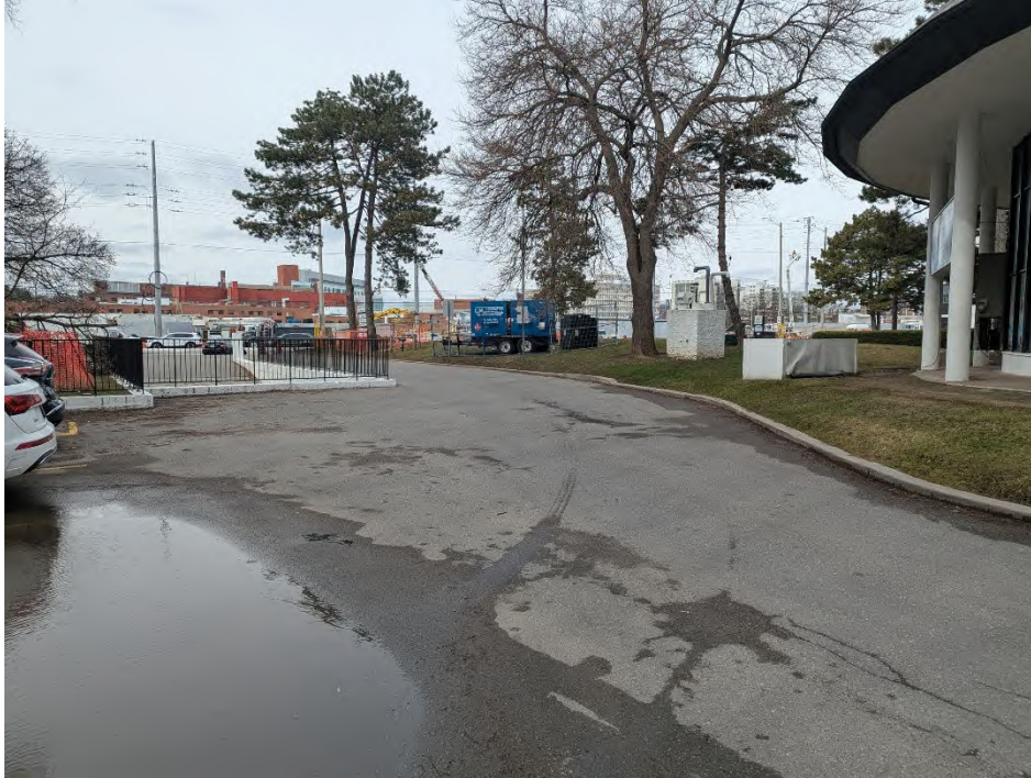
Image 3: View southwest to Hurontario Street in the southwest part of the subject property.
