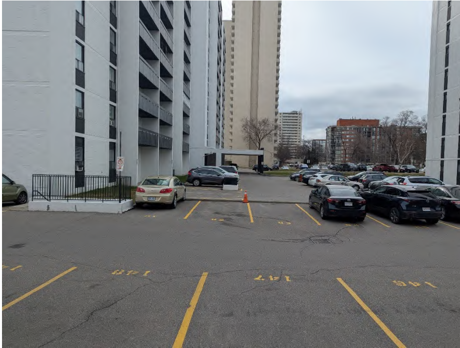
Image 9: View southeast across surface and underground parking to the 2233 building.
