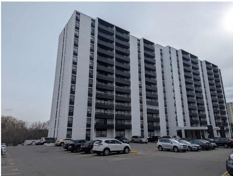
Image 8: View northeast across surface and underground parking to the 2233 building.
