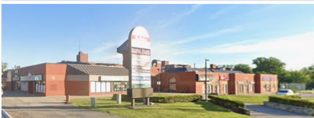
Commercial plaza at northeast of Queensway and Hurontario Street
