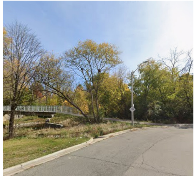
Pedestrian bridge connecting the site to Iggy Kaneff Park.
