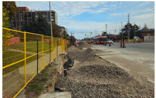
LRT construction looking south along Hurontario Street
