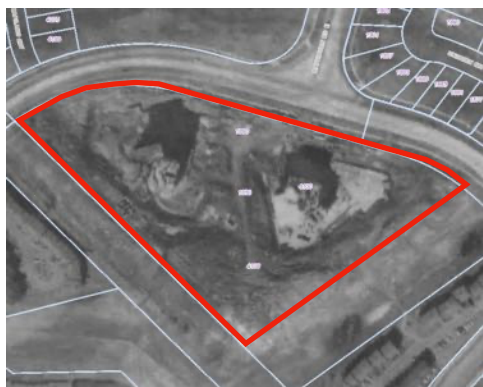
Left: 1980 air photo showing the Study Area, note deep soil excavation, mounding and disturbance from construction.
