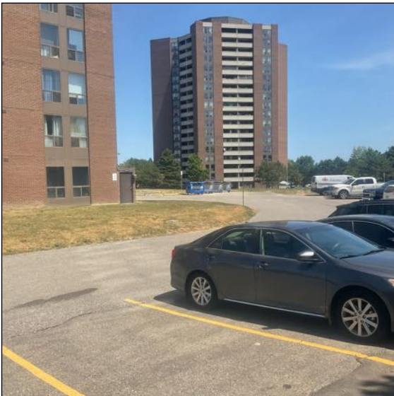
Image 7: View of previously disturbed and graded lands; note structures and utilities.
