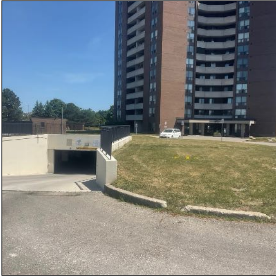
Image 1: View of underground parking entrance and previously disturbed and graded lands.
