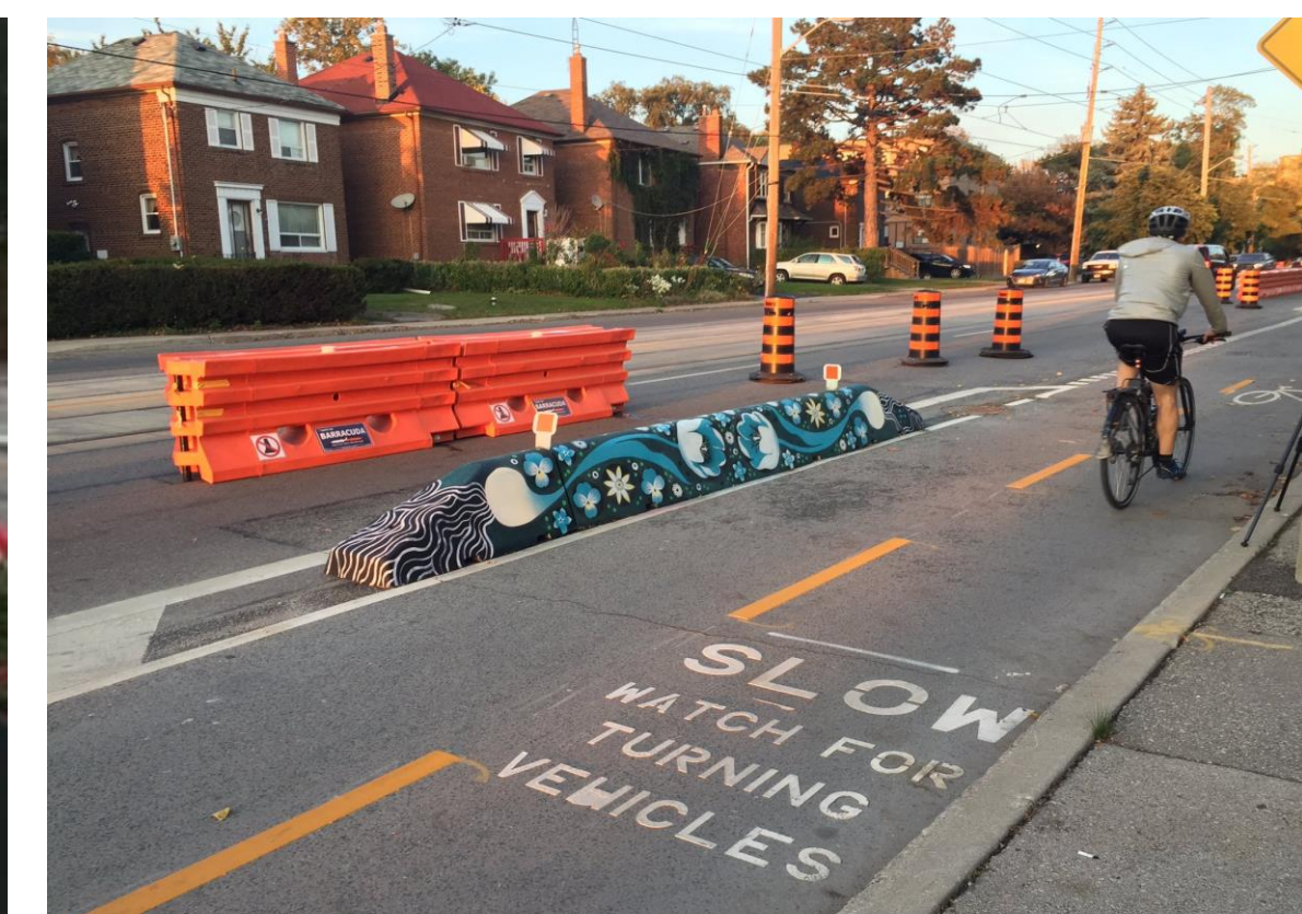
Painted concrete cast curb, modular dividers (orange) and pylons (orange/black)
