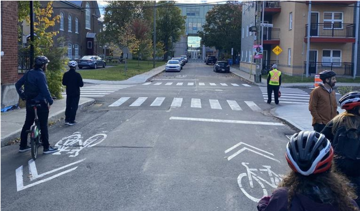
Figure 4.9 An example of "sharrows" on a shared route.
