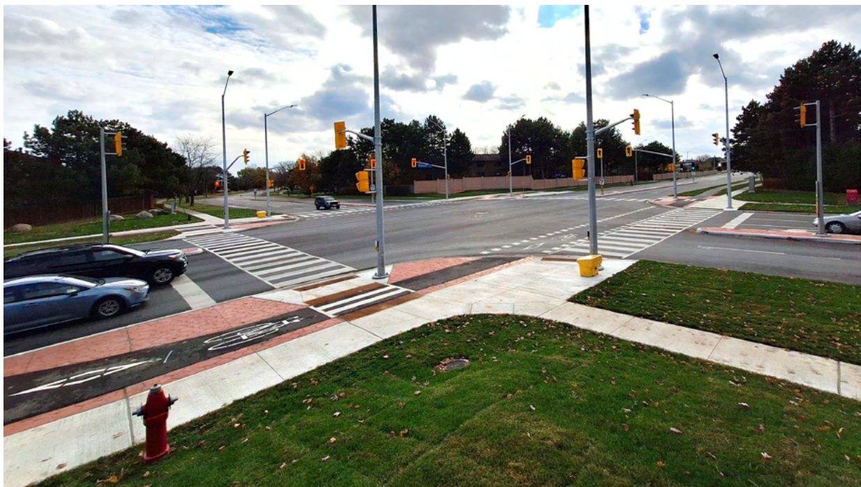
Figure 4.21: Example of a cycle track implemented as part of a larger coordinated roadwork project on Rathburn Road.
