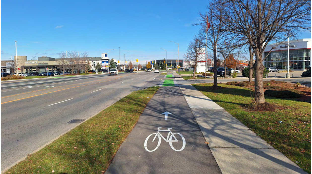
Figure 4.20: Example of a cycle track implemented as a standalone cycling project on Argentia Road.
