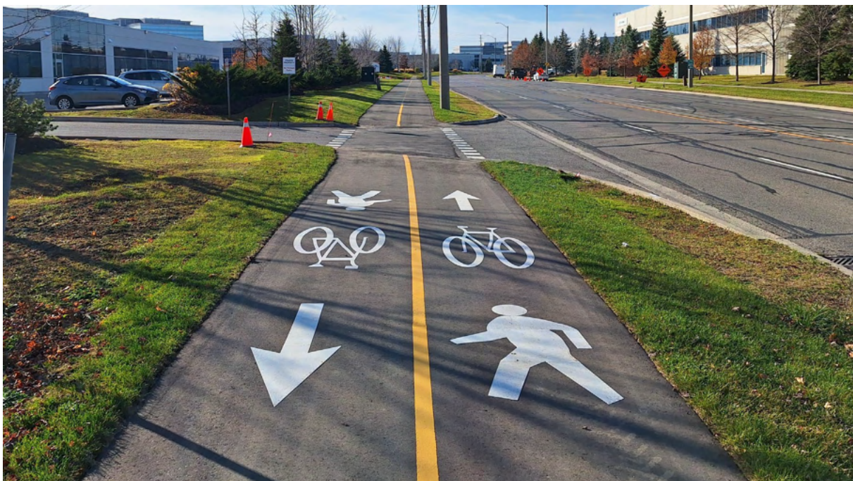
Figure 4.3: A two-way Multi-Use Path that allows for cycling, walking, and rolling in both directions.
