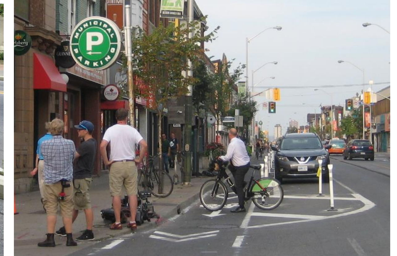
Painted curb extension bollards
