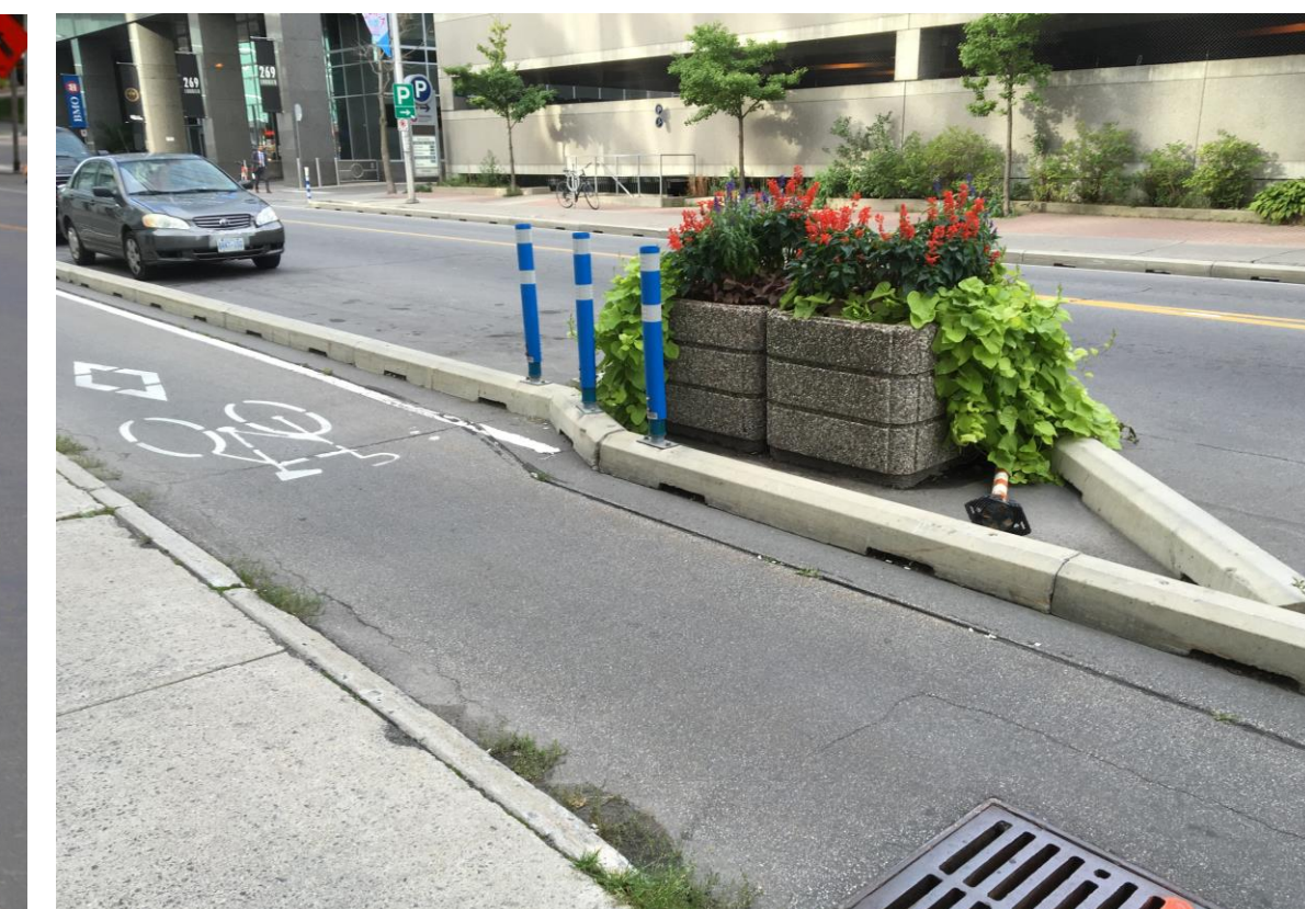
Small modular curb, flexible bollards and planter creating curb extension
