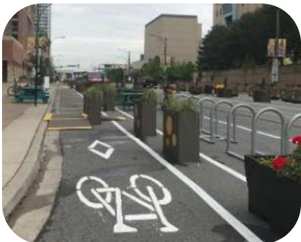
Planters, portable metal bike racks and painted buffer
