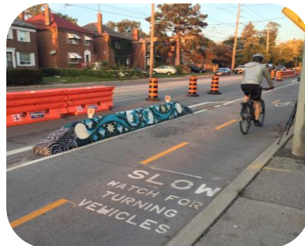
Painted concrete cast curb, modular dividers (orange) and pylons (orange/black)
