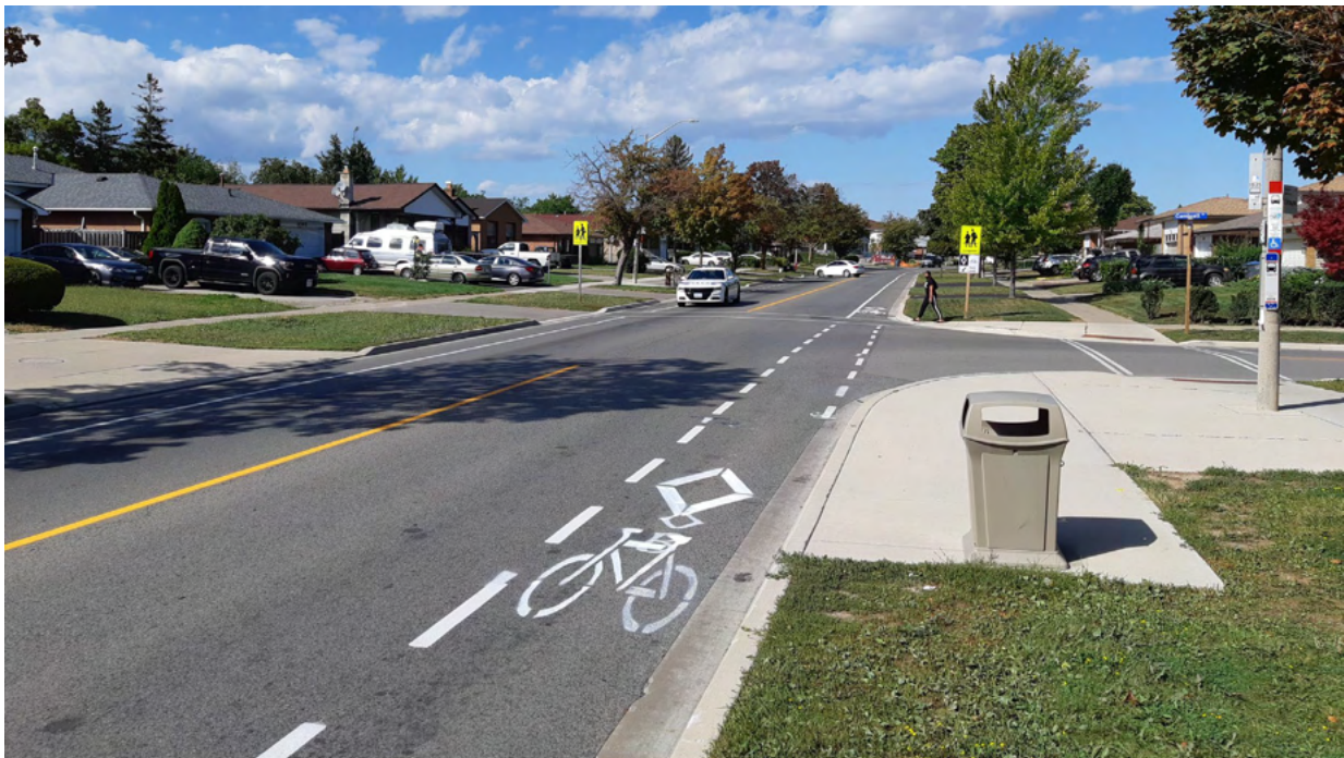
Figure 4.8: Painted (conventional) bike lane on both sides of a two-way road.
