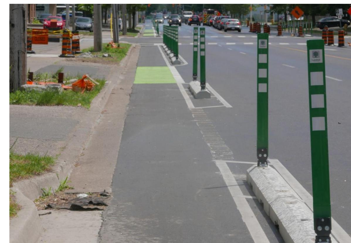
Small concrete curb and flexible bollards
