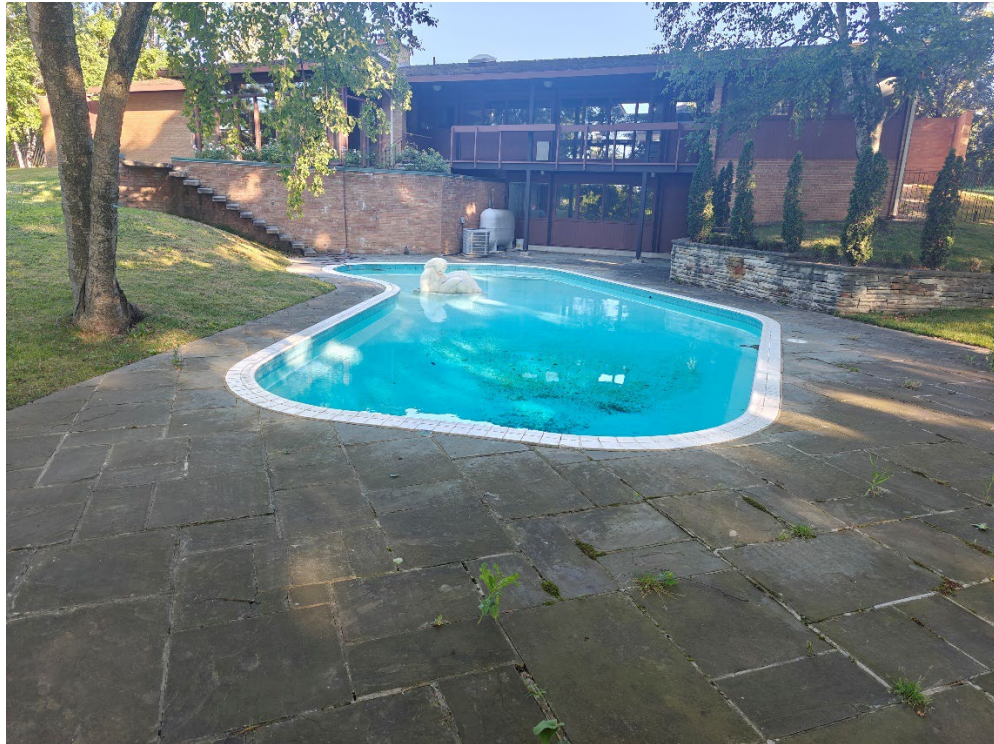
Photo 1: Visible Disturbance Facing North
