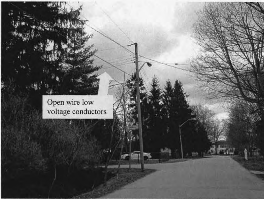
Photograph #5 – Existing low voltage cables with "Open wire configuration"
