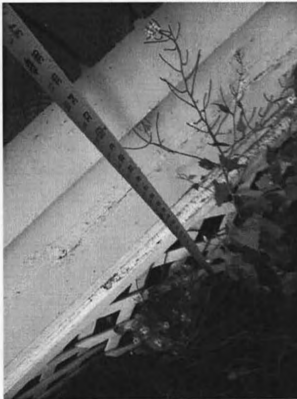
Existing porch showing height
