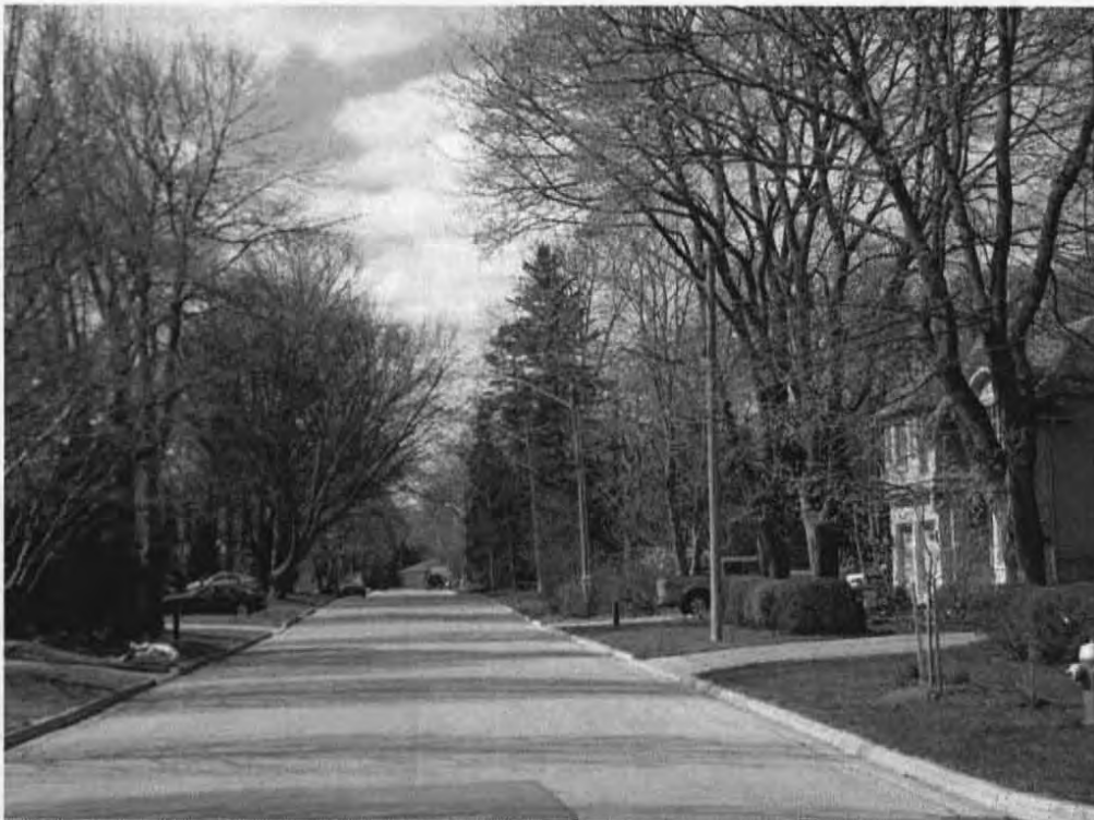
Photograph #2 – Typical Overhead Rebuild in Mississauga with 35 wood poles and low voltage conductors (120/240 V)
