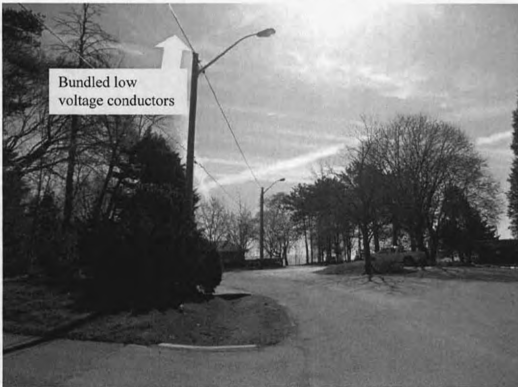
Photograph #6 – New standard with bundled low voltage wires (120/240 V)
