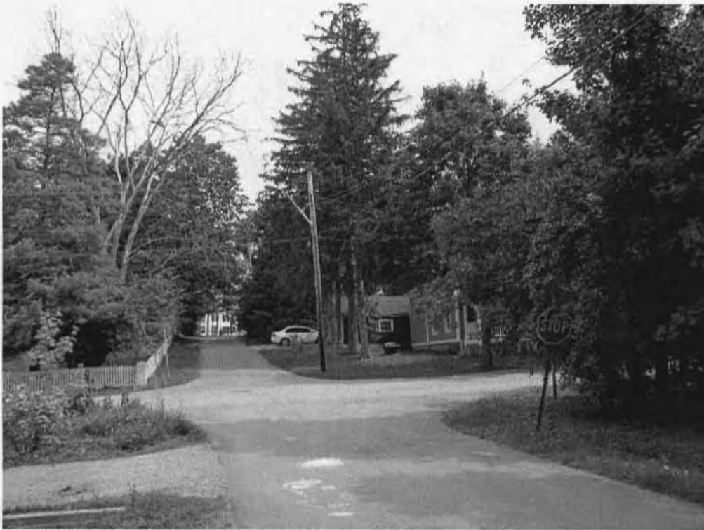
Photograph #1 – Existing 30 foot wood pole on an interior street of Old Meadowvale Village
