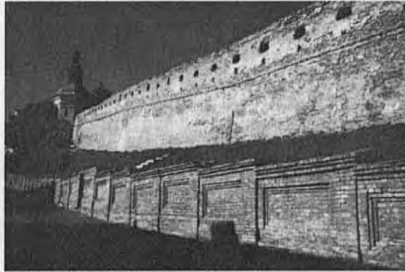
Panelled Wall Relief on Retaining Wall
