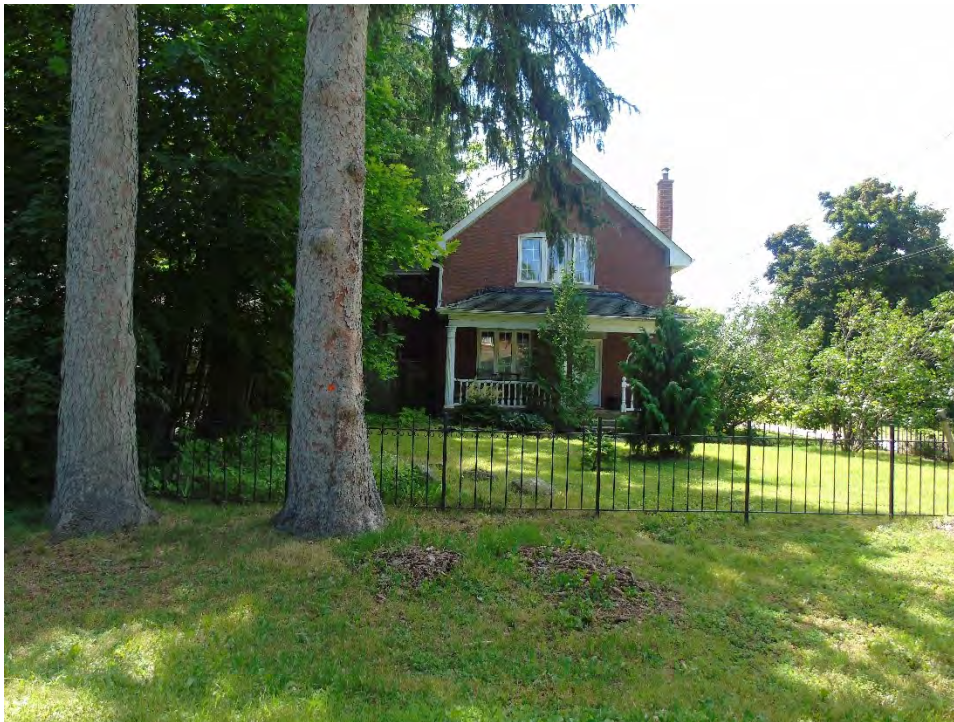
Figure 4-22: Residence in Erindale Village (A.S.I. 2018)
