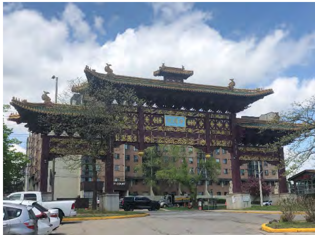
Figure 11 Existing Entrance Gate to 888 Dundas Street East
