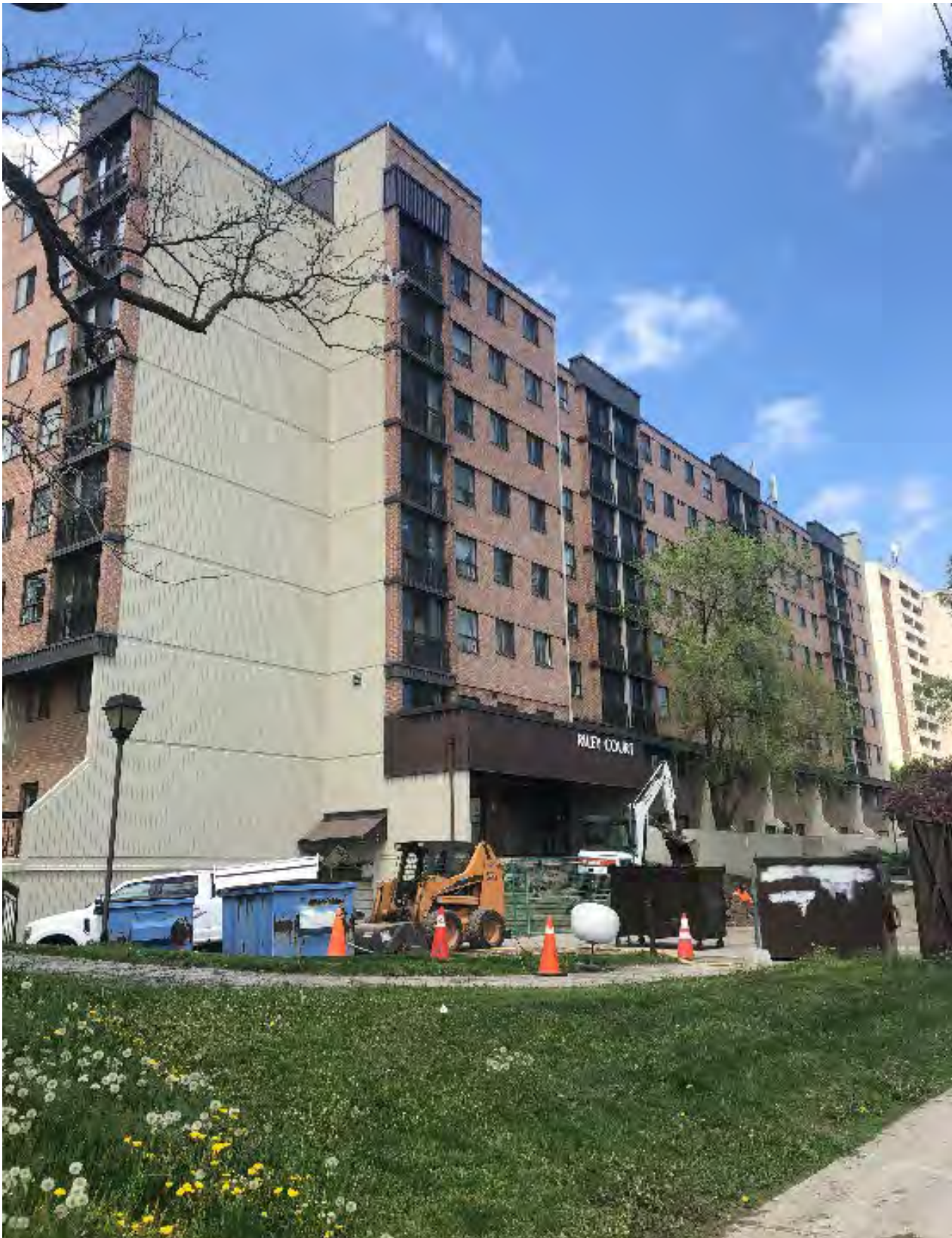
Figure 9-Existing 8 storey apartment building at 888 Riley Court
