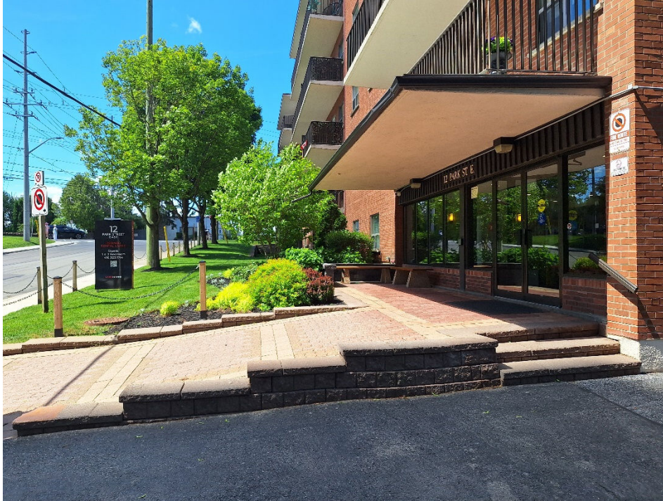
Image 2: View west across the front of the 12 Park apartment building.
