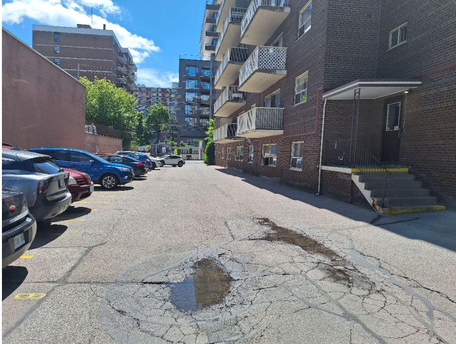
Image 14: View south southeast along the driveway to the 26 Park parking lot.
