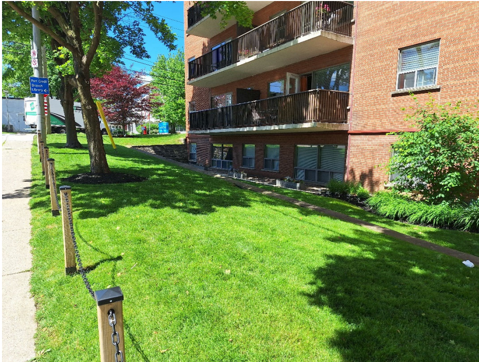
Image 1: View west to the southwest corner of the 12 Park apartment building.
