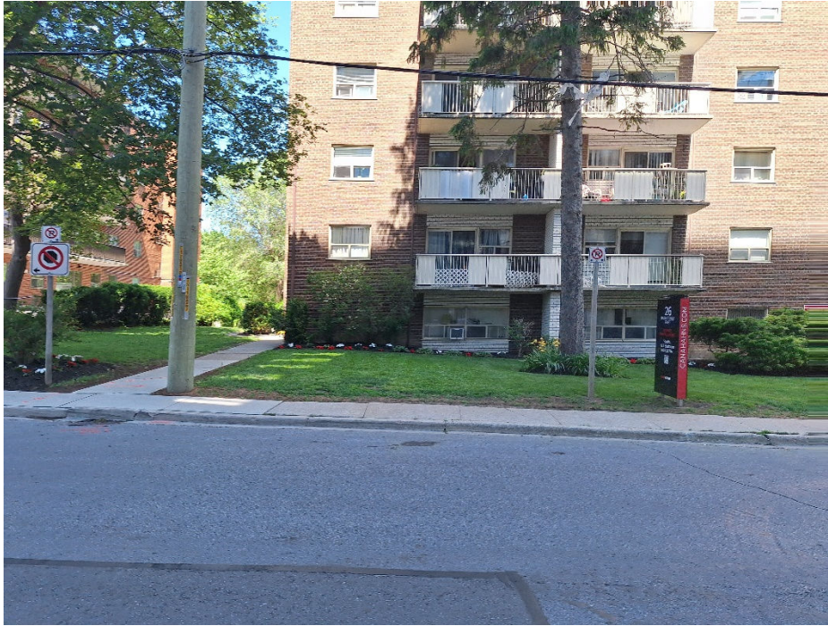
Image 4: View northwest to the front of the 26 Park apartment building.
