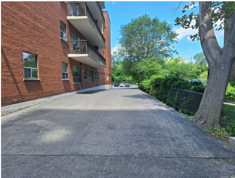
Image 3: View northwest along the 12 Park driveway to the rear parking lot.
