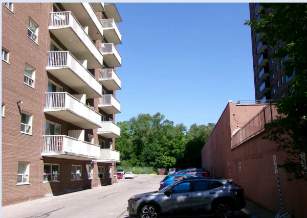
1. Drive Aisle Along the East Property Line
