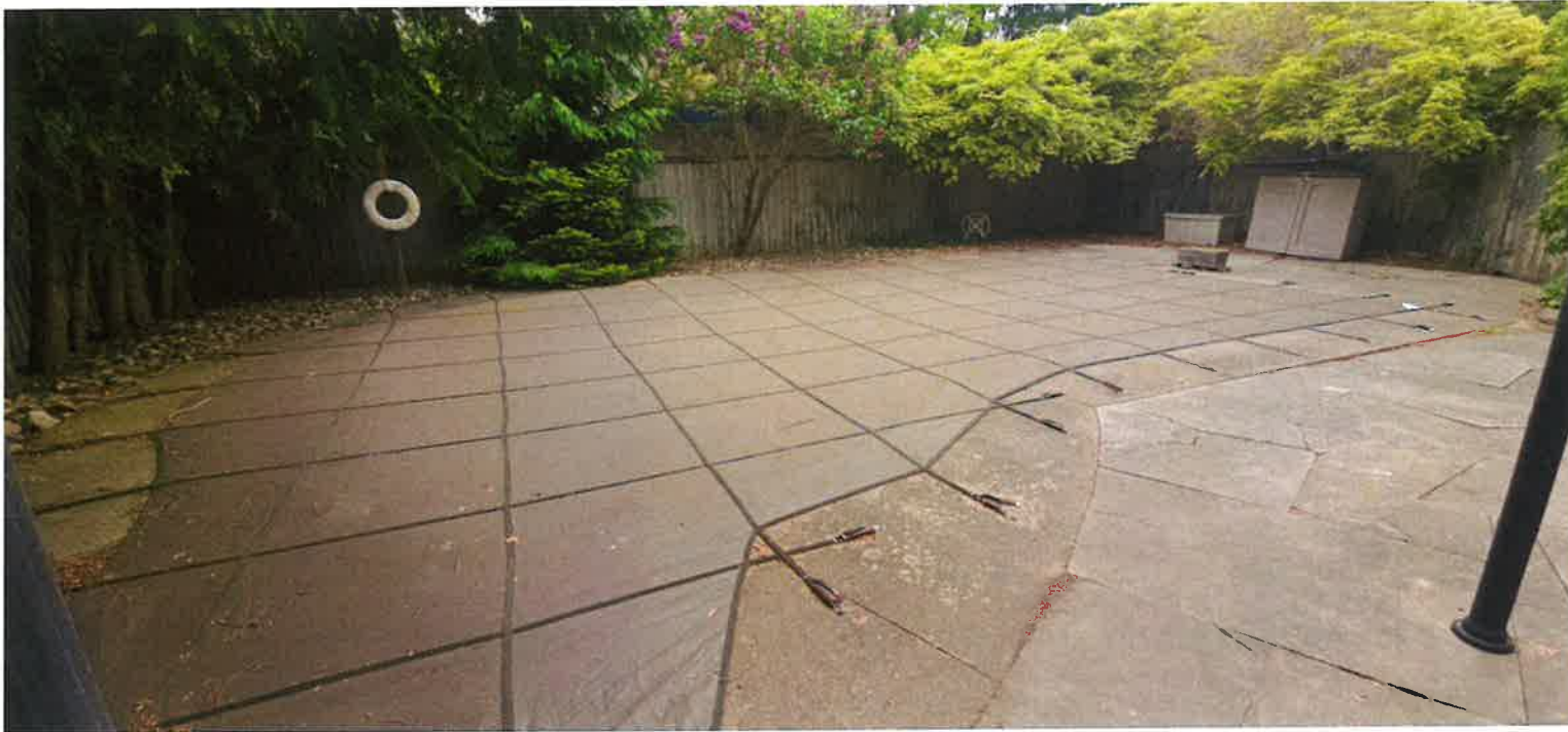
General view of the covered outdoor pool located south of the residential building (looking south)
