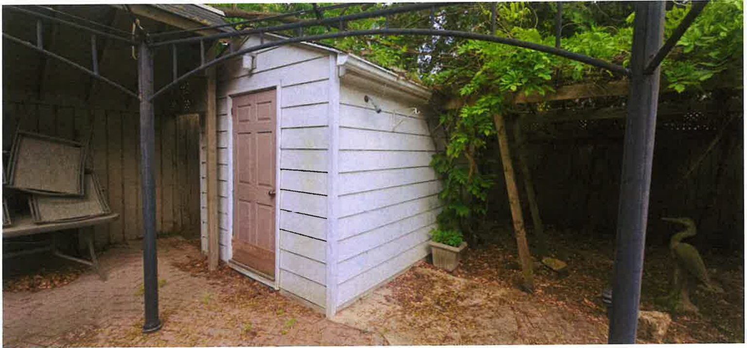
General view of the second shed located east of the residential building (looking east)
