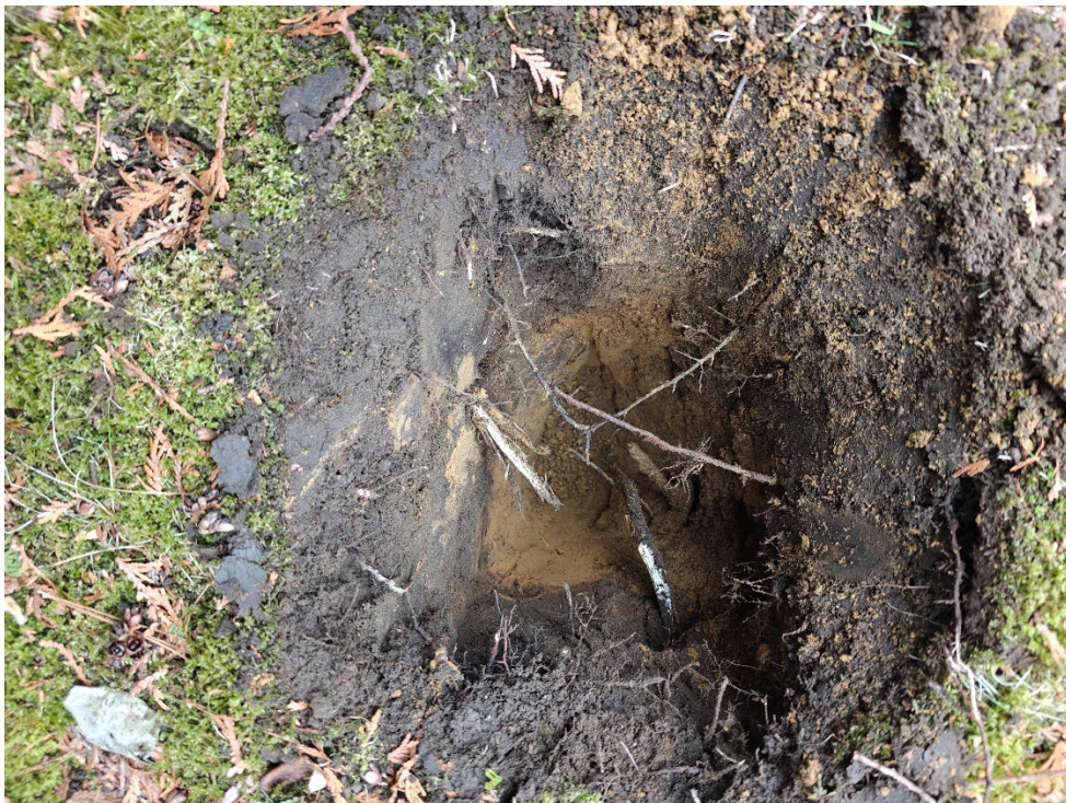
Photo 8: Typical Test Pit Facing West
