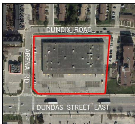
Aerial image of 1225 Dundas Street East
