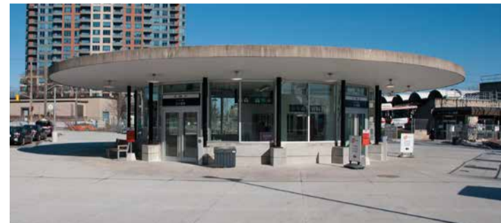
Accessible Pedestrian Tunnel to TTC Kipling Station
