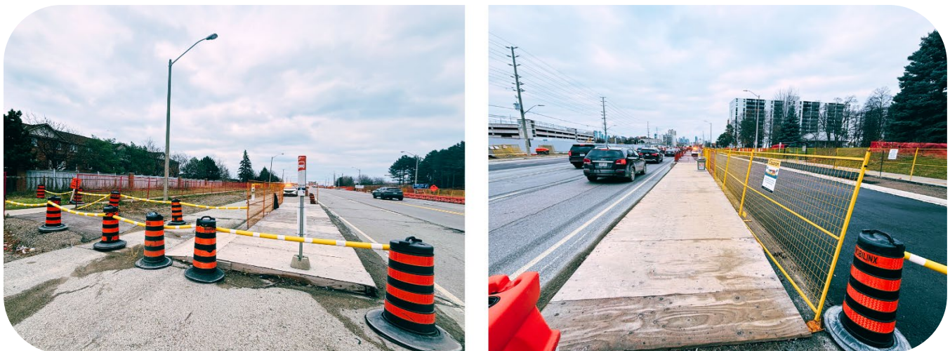
Figure 7: Temporary pedestrian walkways and ramps.
