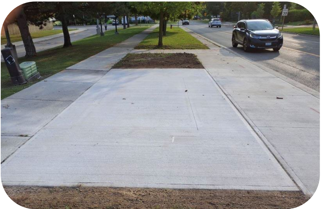
Figure 4: New customer landing pad and shelter pad at bus stop #0122 Bromsgrove Road at Playford Road.
