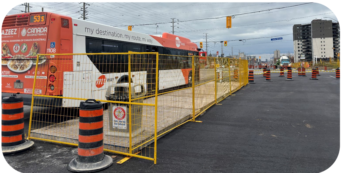
Figure 9: Temporary pedestrian landing pad platform.
