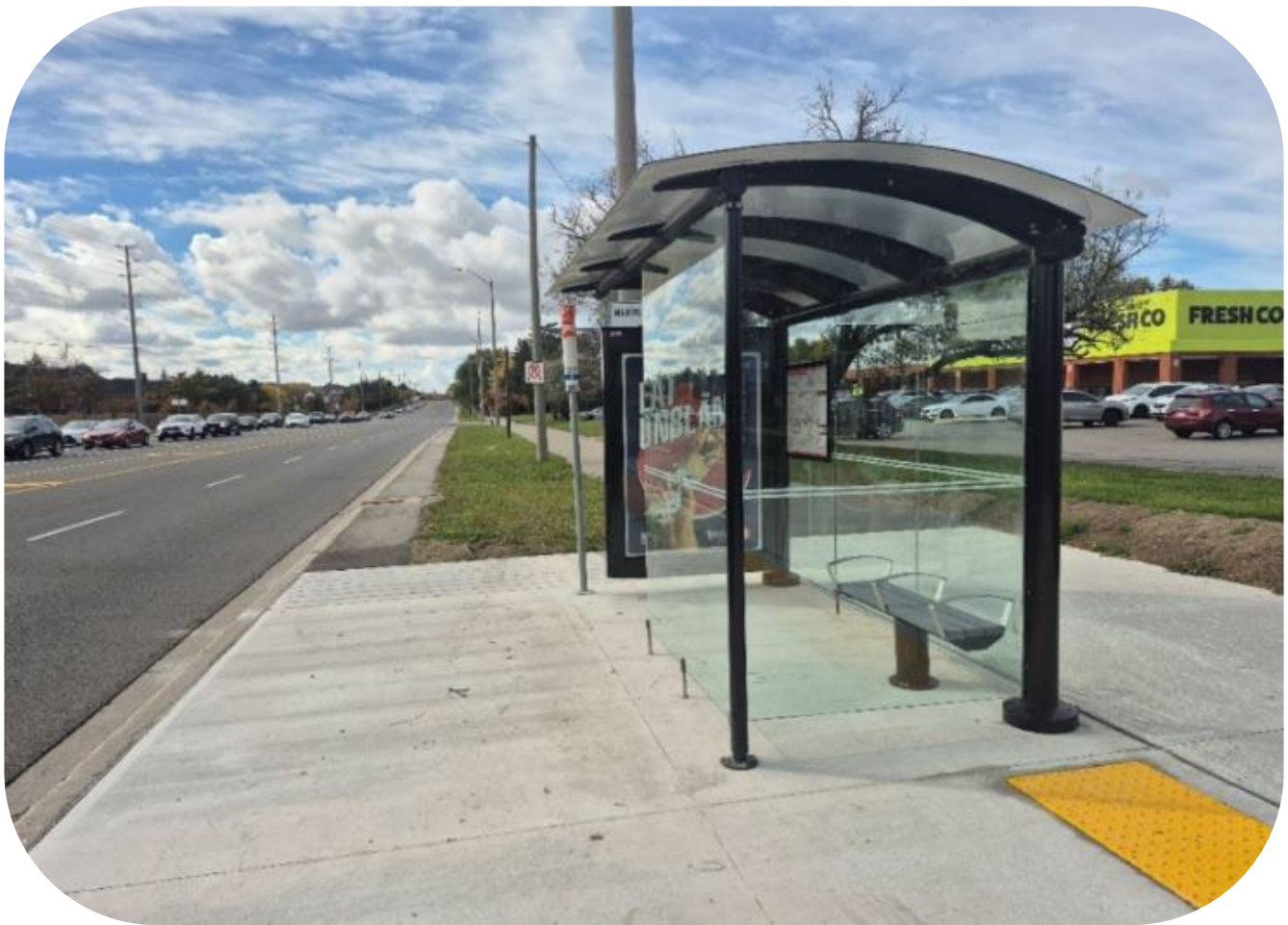
Figure 6: Example at mixing zone improvement at stop #1887 Britannia Road and Glen Erin Drive
