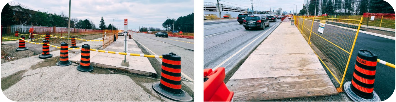
Figure 10: Temporary pedestrian walkways and ramps.
