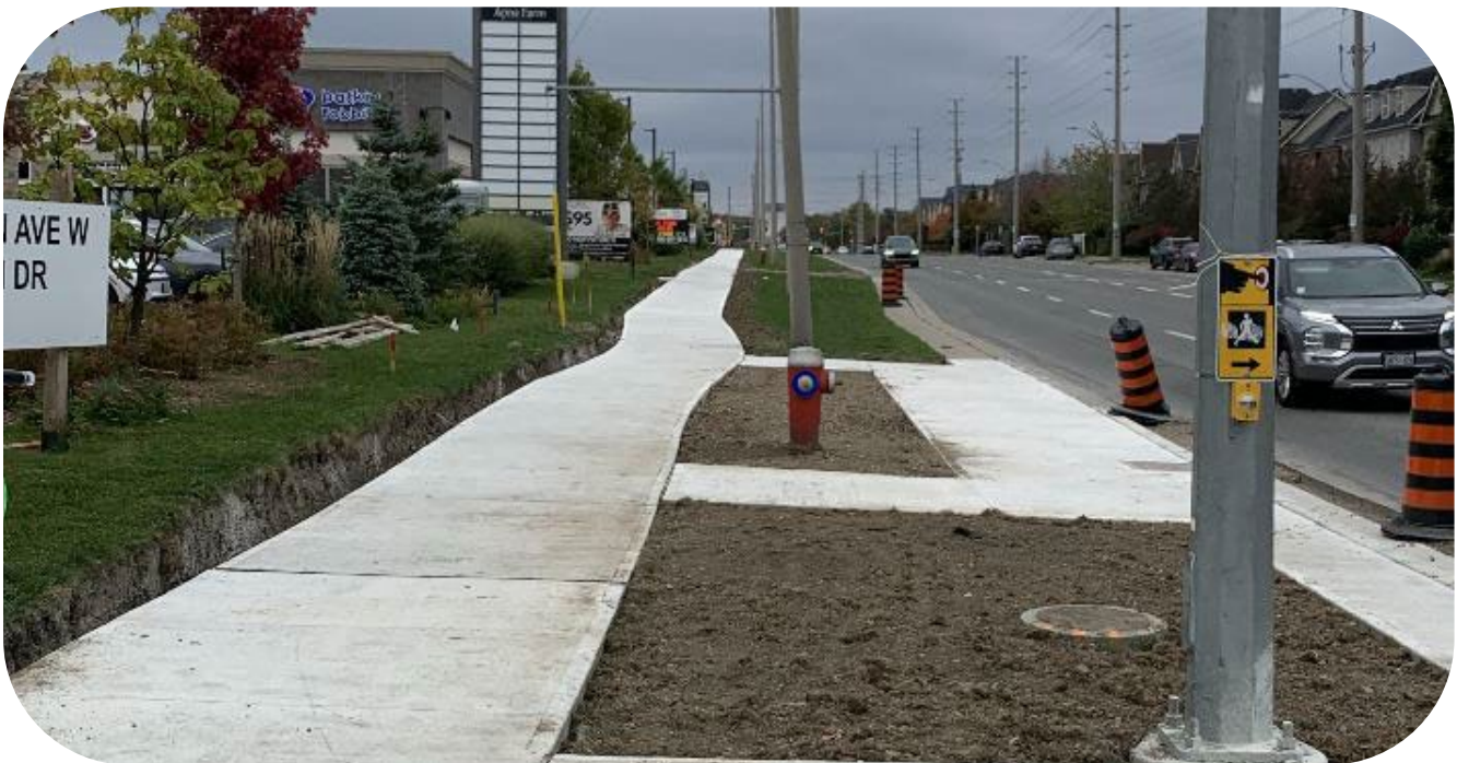
Figure 7: New Stop Infrastructure on Eglinton Ave in 2025 Sidewalk Program
